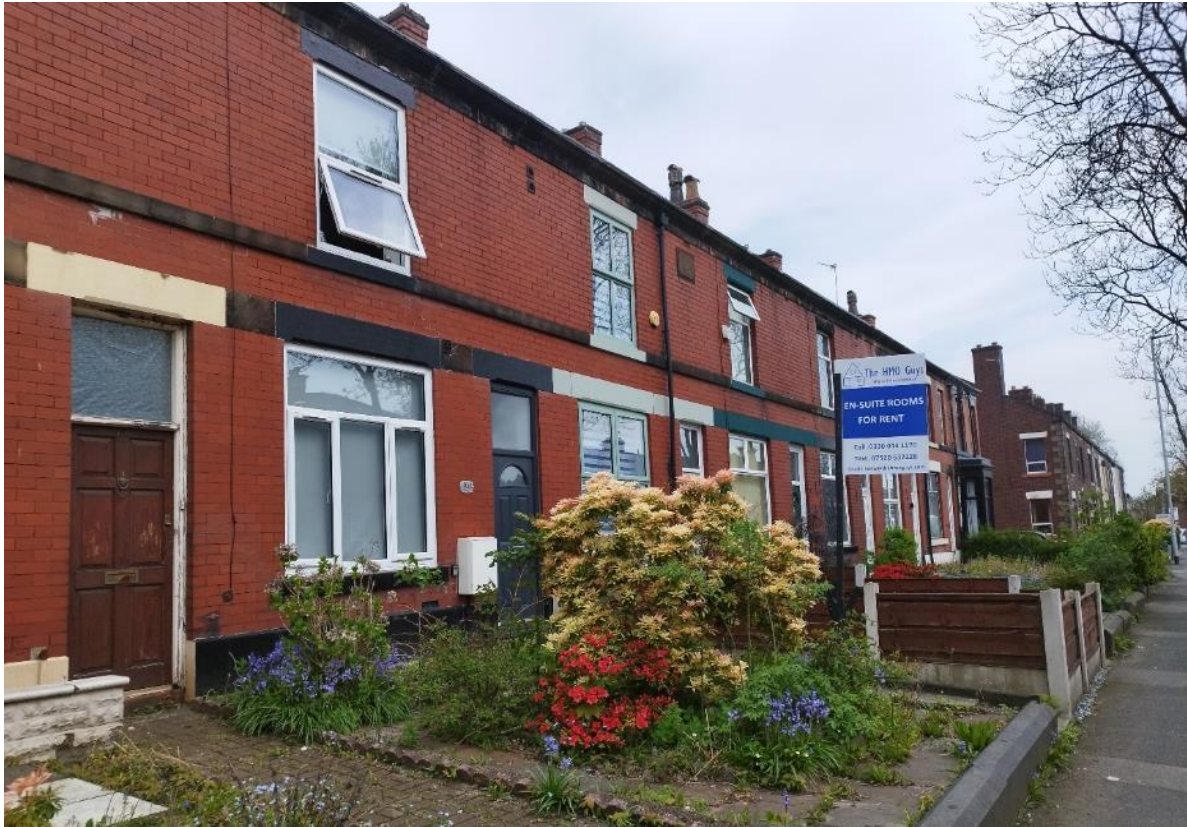
Frontage of 104 Ainsworth Road
