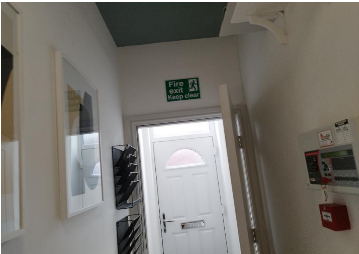
Front doorway and hallway at 104 Ainsworth Road
