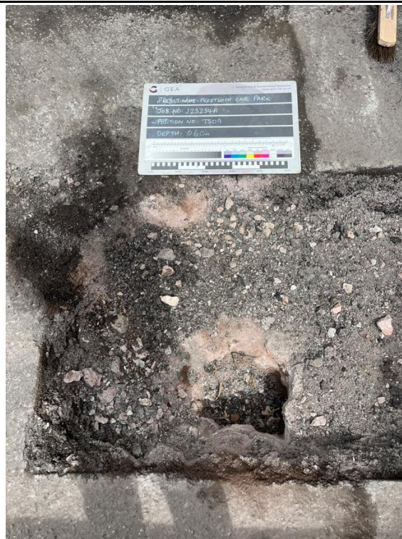
TS09 - Excavation locally to a depth of 0.60 m looking northwest
