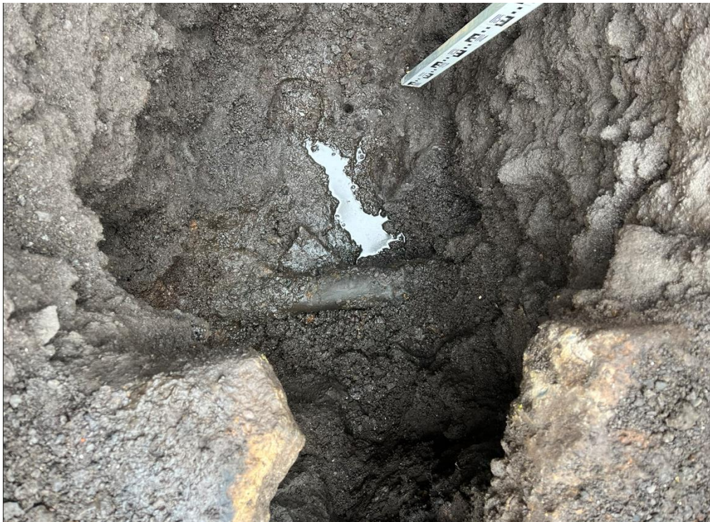
TS03 - Cast iron pipe at base of the excavation
