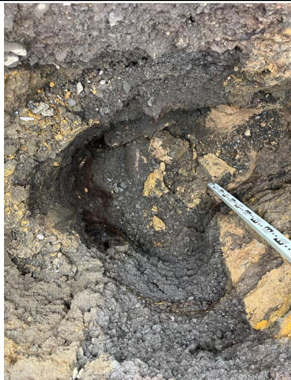
TS04 - Closer view of drainage pipe
