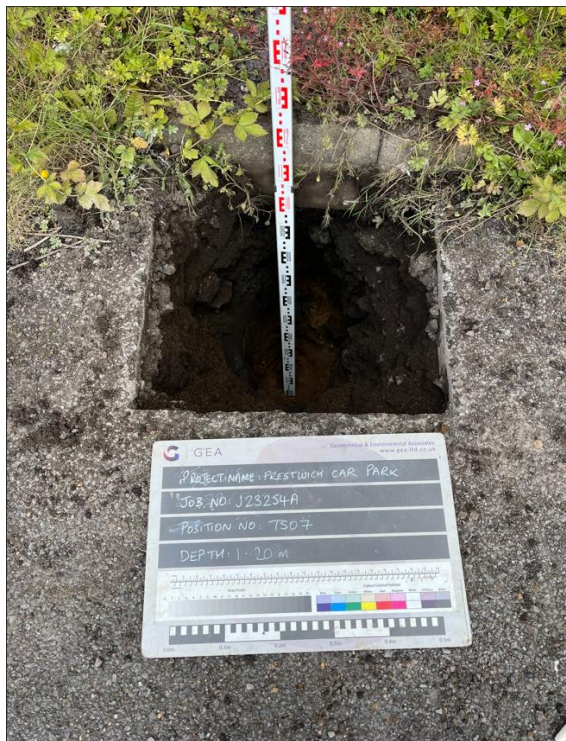
TS07 - Excavation to a depth of 1.20 m looking northwest - no services encountered
