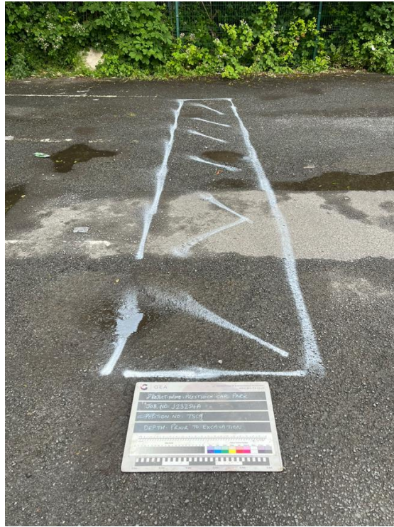
TS09 - Prior to excavation looking northeast
