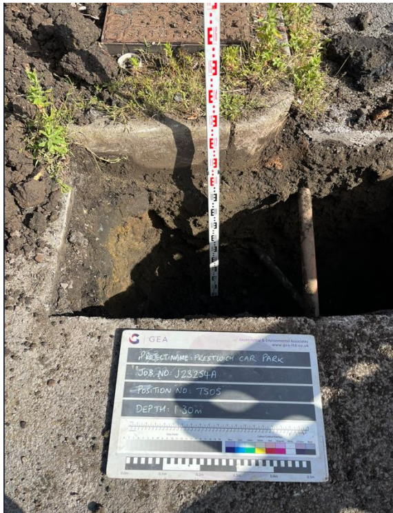
TS05 - Excavation to a depth of 1.30 m looking northwest - low voltage electric and BT ducts encountered
