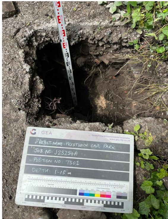
TS02 - Excavation to a depth of 1.15 m looking northwest - no services encountered
