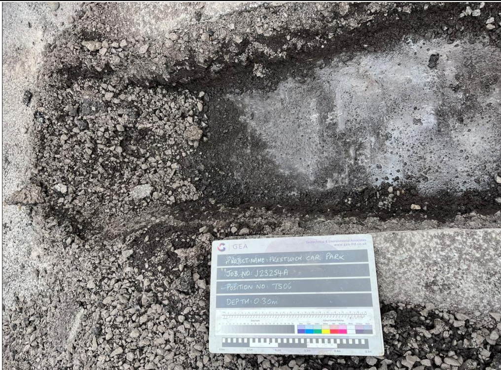
TS06 - Excavation to a depth of 0.30 m looking southwest - concrete encountered
