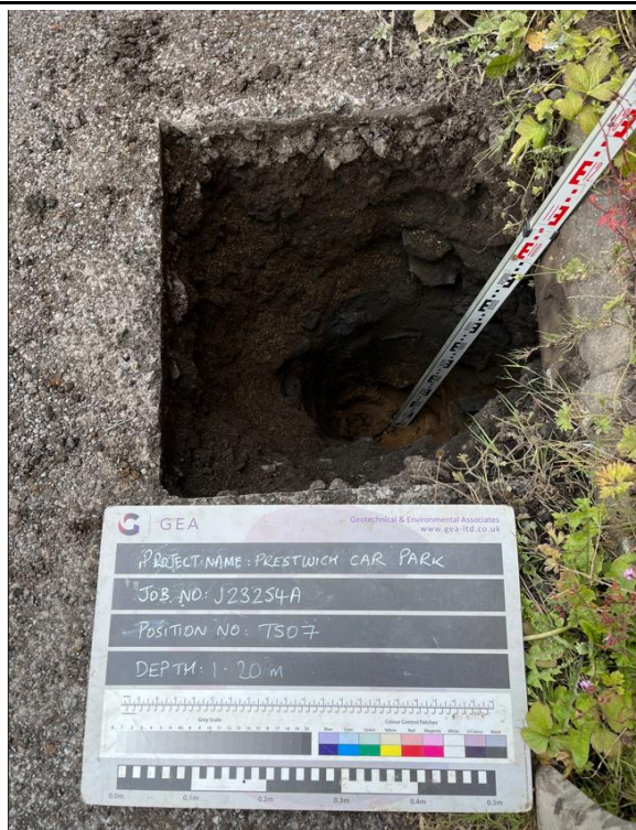
TS07 - Excavation to a depth of 1.20 m looking southwest - no services encountered
