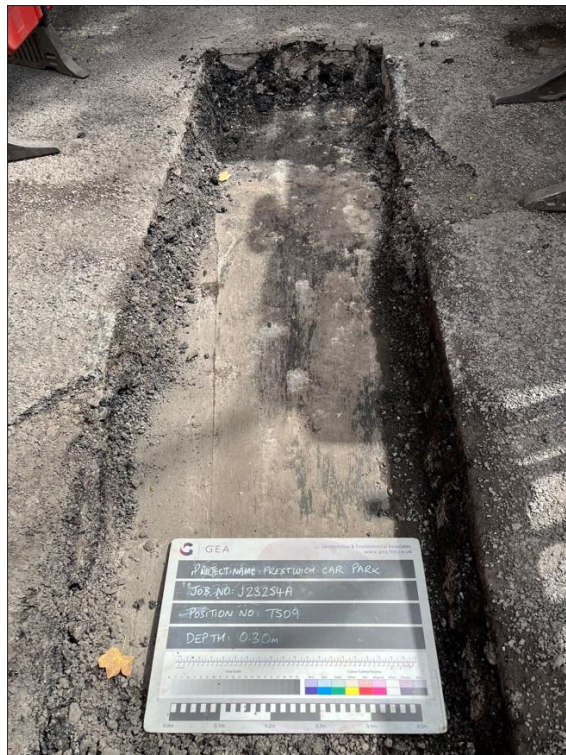
TS09 - Excavation to a depth of 0.30 m looking northeast - concrete encountered
