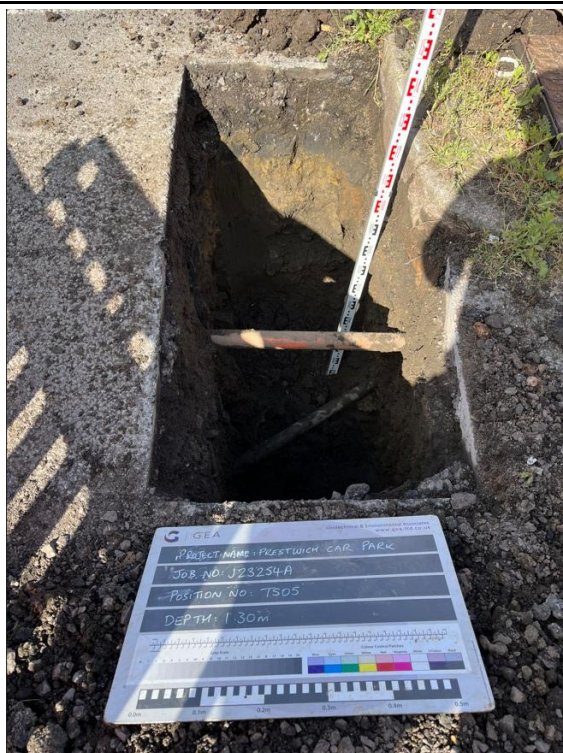
TS05 - Excavation to a depth of 1.30 m looking southwest - low voltage electric and BT ducts encountered
