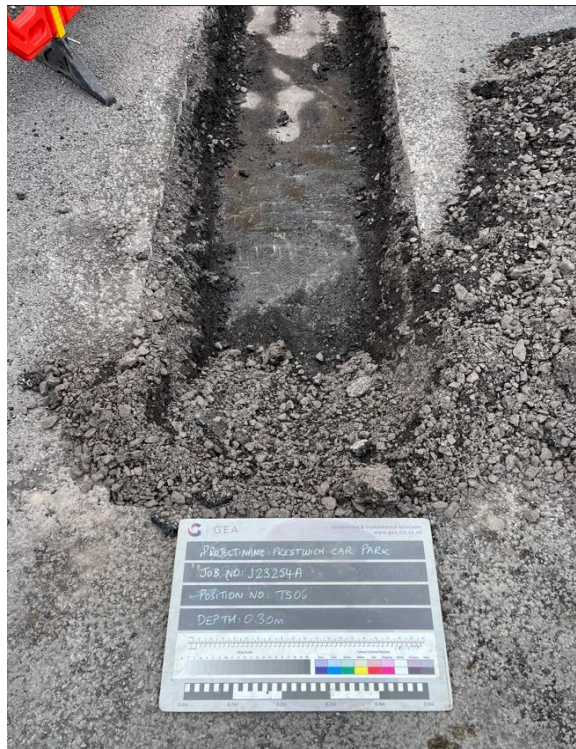
TS06 - Excavation to a depth of 0.30 m looking northwest - concrete encountered
