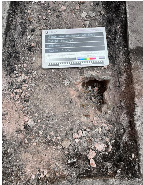
TS09 - Excavation locally to a depth of 0.60 m looking northeast
