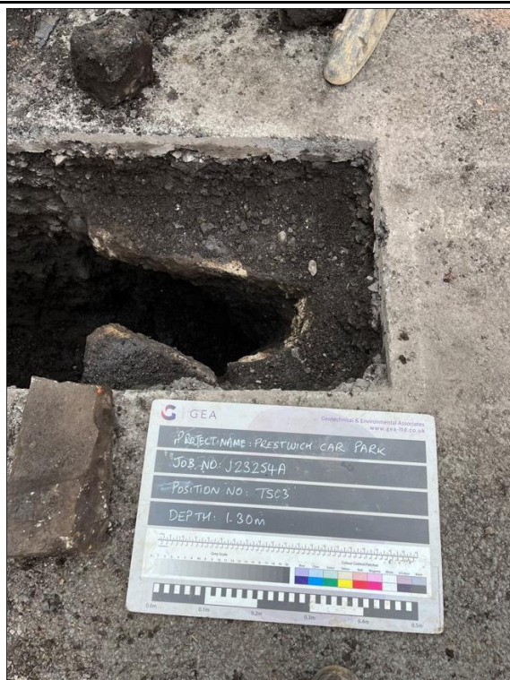
TS03 - Excavation to a depth of 1.30 m looking southeast
