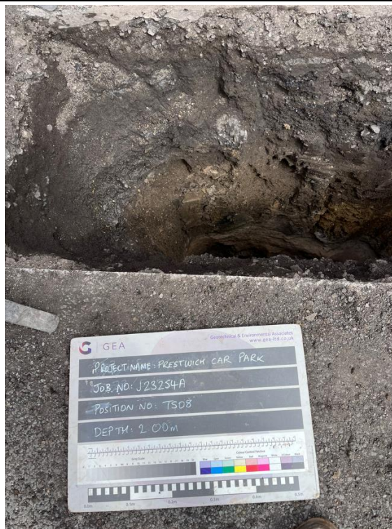
TS08 - Excavation to a depth of 2.00 m looking northwest - no services encountered
