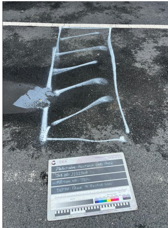
TS04 - Prior to excavation looking northeast
