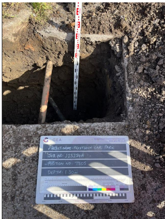
TS05 - Excavation to a depth of 1.30 m looking northwest - low voltage electric and BT ducts encountered
