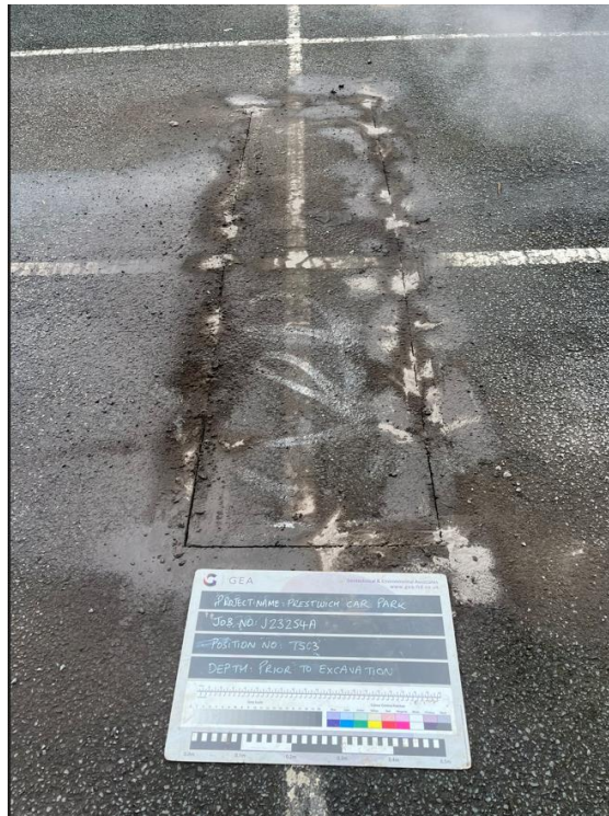
TS03 - Prior to excavation looking northeast
