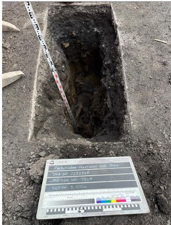
TS08 - Excavation to a depth of 2.00 m looking southwest - no services encountered
