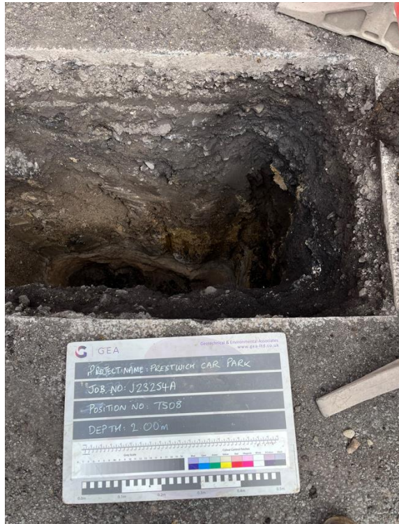
TS08 - Excavation to a depth of 2.00 m looking northwest - no services encountered
