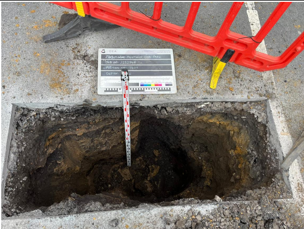
TS04 - Excavation to a depth of 1.80 m looking southeast - drainage pipe encountered
