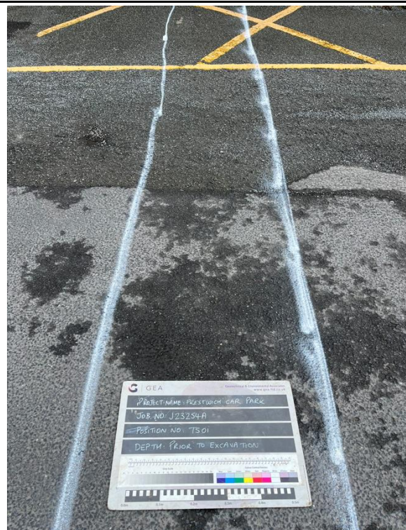
TS01 - Prior to excavation looking southwest
