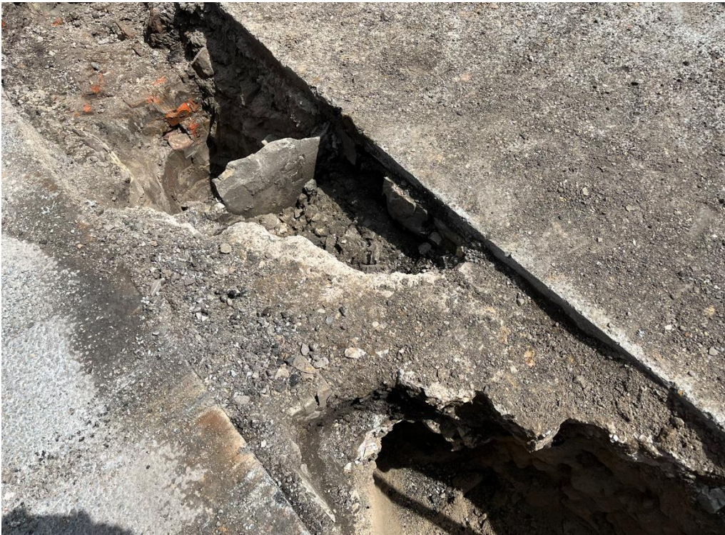
TS01 - Layer of concrete atop a shallow drainpipe within the central part of the excavation
