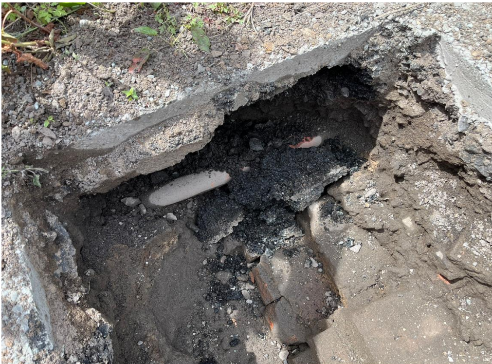
TS01 - Orange duct within the western part of the excavation
