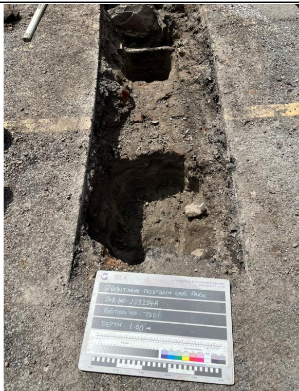
TS01 - Eastern part of the excavation to a depth of 1.00 m looking southwest
