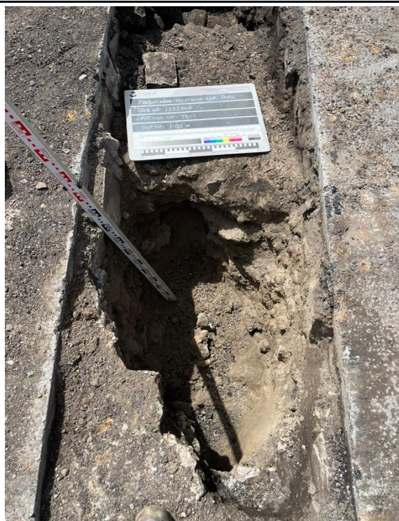
TS01 - Central part of the excavation to a depth of 1.00 m looking southwest.
