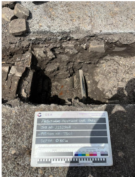
TS01 - Central part of the excavation to a depth of 0.85 m looking northwest containing drainage pipe and a black duct
