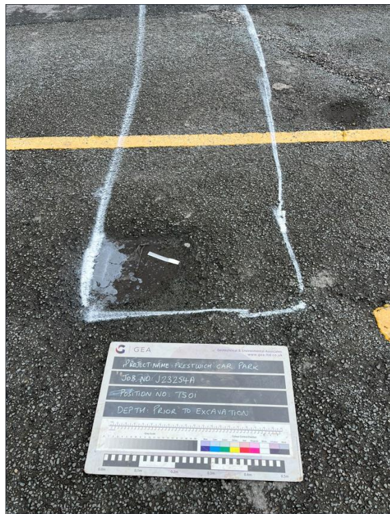
TS01 - Prior to excavation looking southwest
