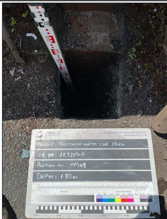
TP103 - Excavation to a depth of 1.70 m looking northeast.
