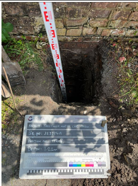
TP104 - Excavation to a depth of 1.26 m looking southeast.
