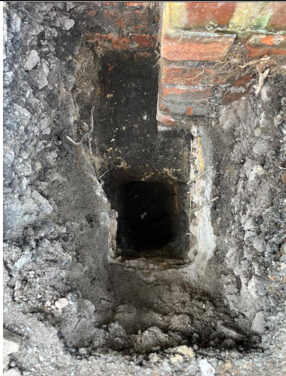
TP105 - Closer view of foundation
