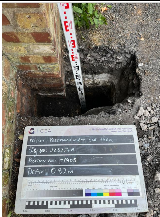
TP105 - Excavation to a depth of 0.82 m looking northwest.
