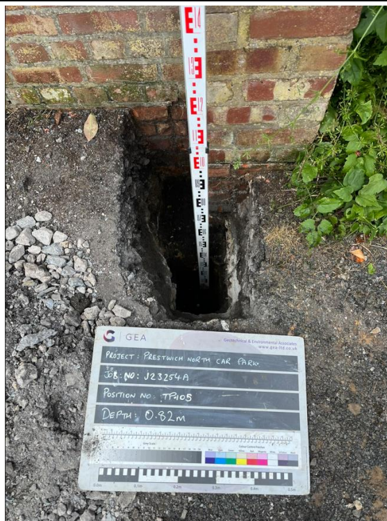
TP105 - Excavation to a depth of 0.82 m looking southwest.
