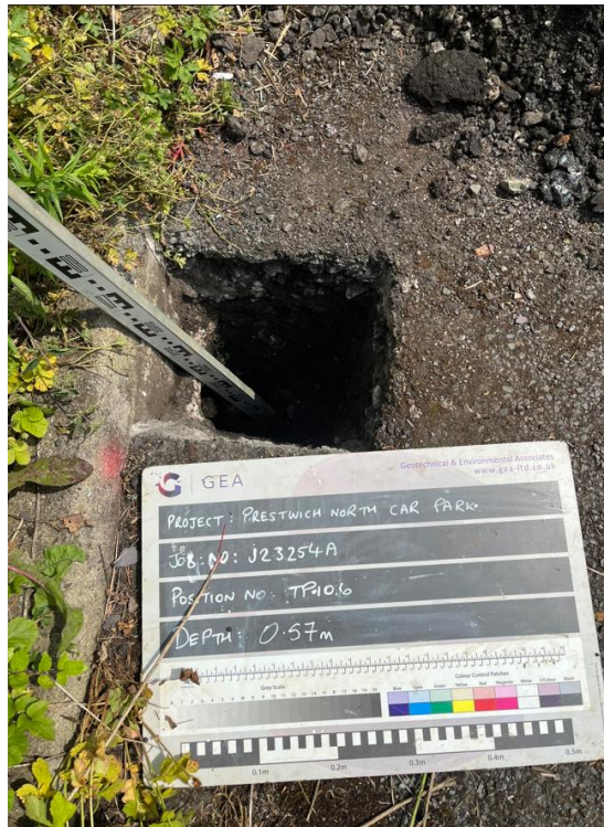
TP106 - Excavation to a depth of 0.57 m looking northeast.
