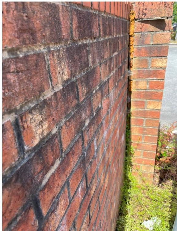
TP103 - Join between brick wall and column located close the position infilled with orange insulation foam
