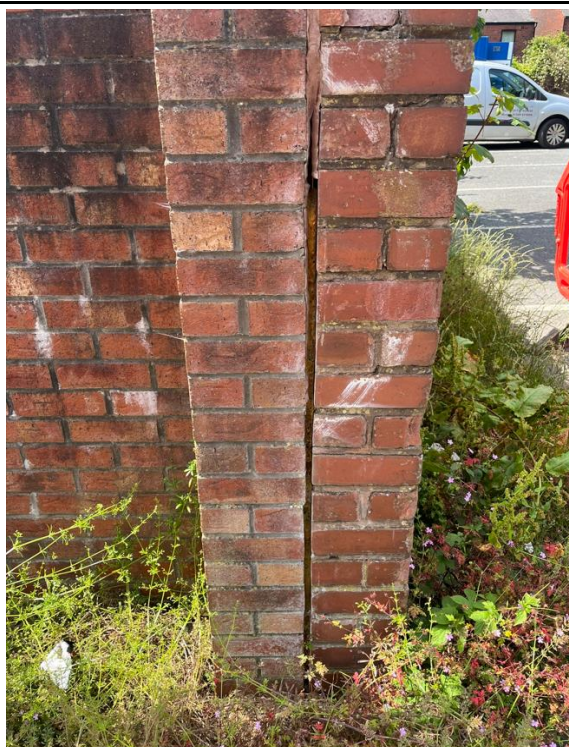
TP103 - Join between brick columns located close the position infilled with orange insulation foam
