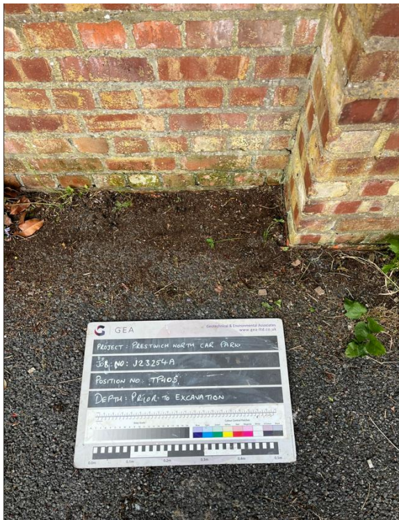
TP105 - Prior to excavation looking southwest.
