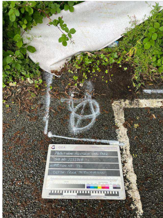
TS11 - Prior to excavation looking northeast
