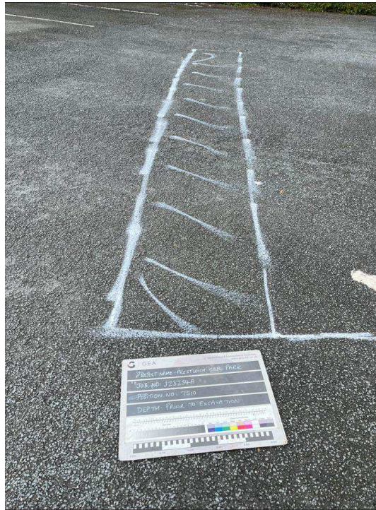
TS10 - Prior to excavation looking northeast
