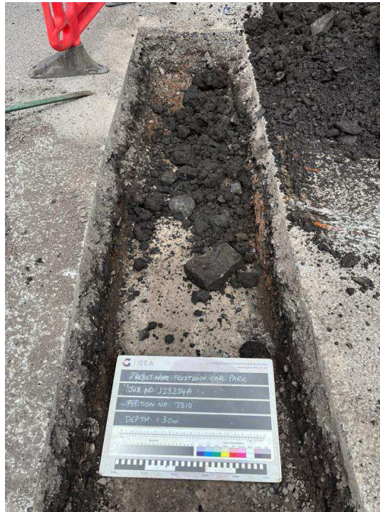
TS10 - Excavation to a depth of 1.30 m looking northeast - concrete encountered
