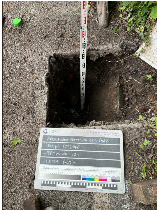
TS11 - Excavation to a depth of 1.00 m looking northwest - no services encountered
