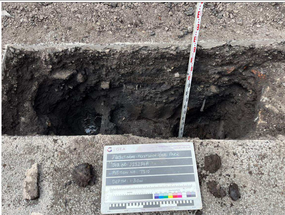
TS10 - Excavation to a depth of 1.30 m looking northwest - cast iron pipe and BT duct encountered
