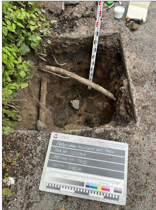
TS12 - Excavation to a depth of 1.00 m looking northwest - low voltage and BT duct encountered
