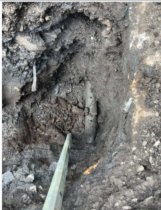
TS10 - Closer view of cast iron pipe
