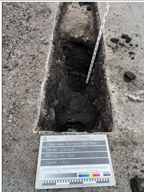
TS10 - Excavation to a depth of 1.30 m looking northeast - cast iron pipe and BT duct encountered
