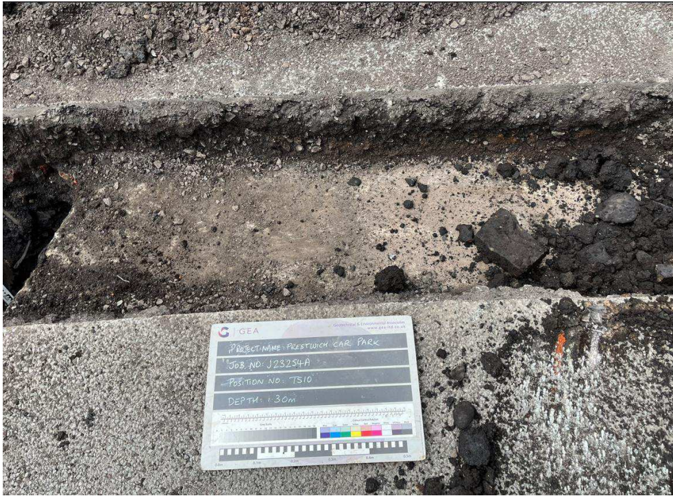
TS10 - Excavation to a depth of 1.30 m looking northwest - concrete encountered
