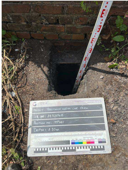
TP101 - Excavation to a depth of 1.30 m looking southwest
