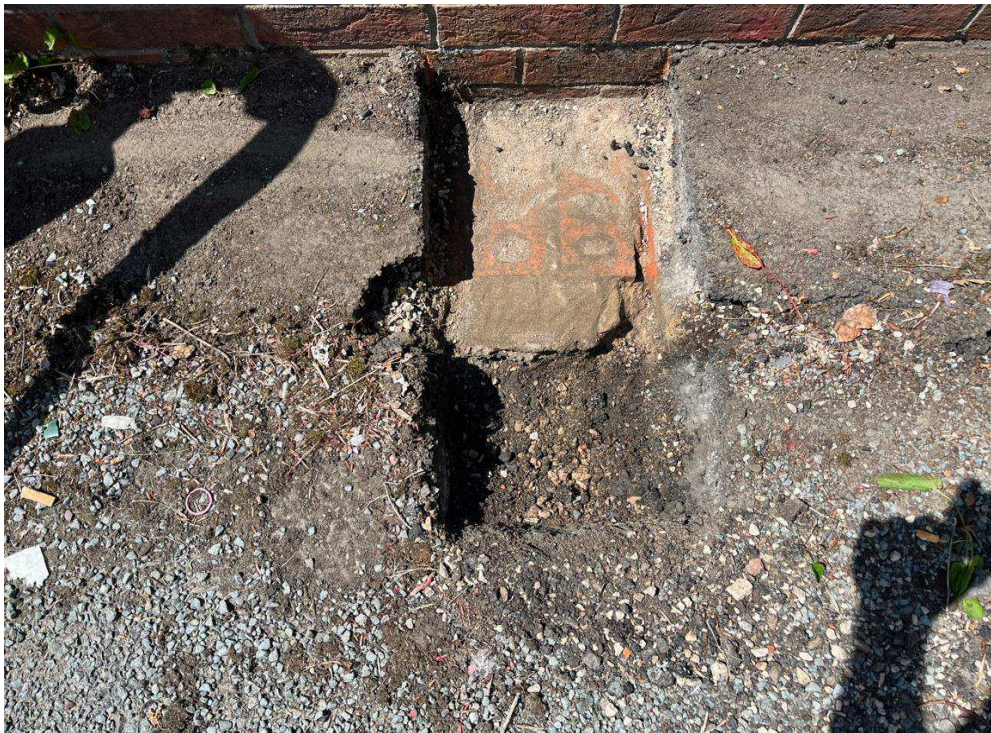
TP102 - View of footing
