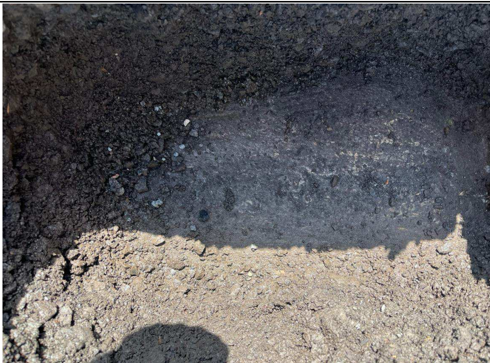
TP102 - Closer view of concrete slab
