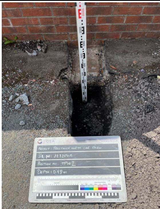
TP102 - Excavation to a depth of 0.48 m looking southwest.
