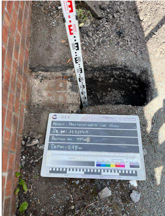
TP102 - Excavation to a depth of 0.48 m looking northeast.
