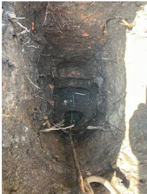
TP101 - Closer view of foundation
