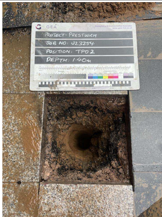
TP02 - Excavated to 1.40 m, looking south
