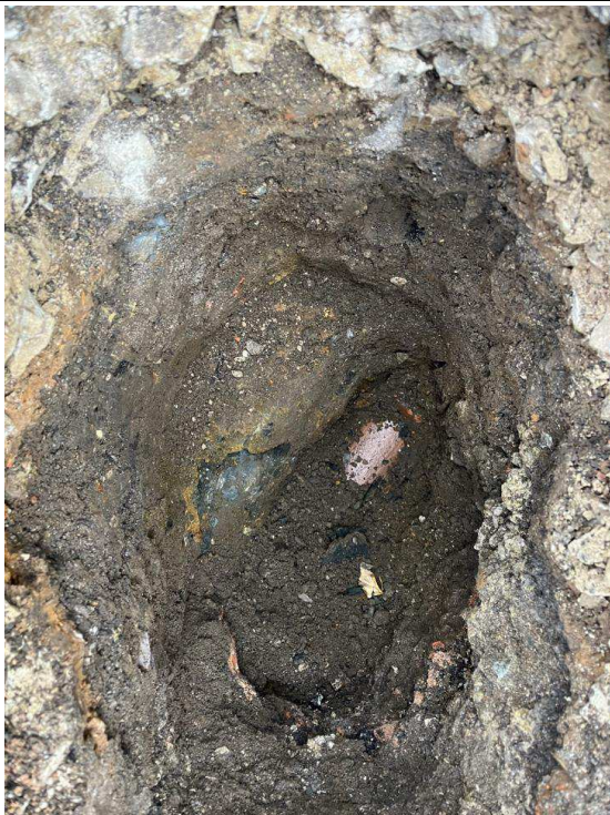
TP04 - Possible gas main and drainage pipe
