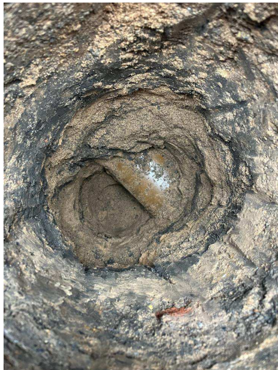
TP03 - Drainage pipe at 1.15 m
