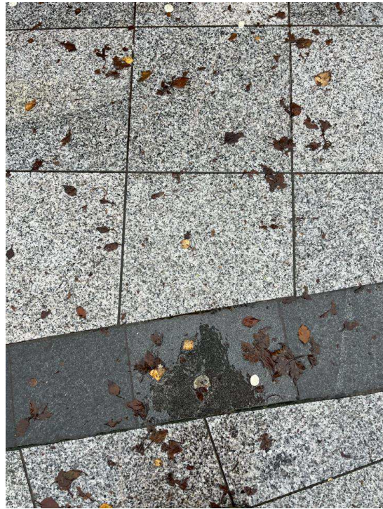
TP04 - Prior to excavation
