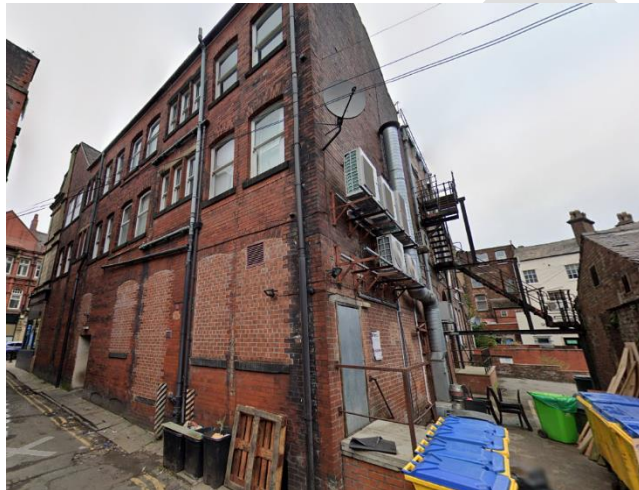
Pic 3 shows the view looking north across Back Broad Street towards the southern side and rear elevations of Victoria Buildings (August 2020). The fire escape etc., has since been removed.
