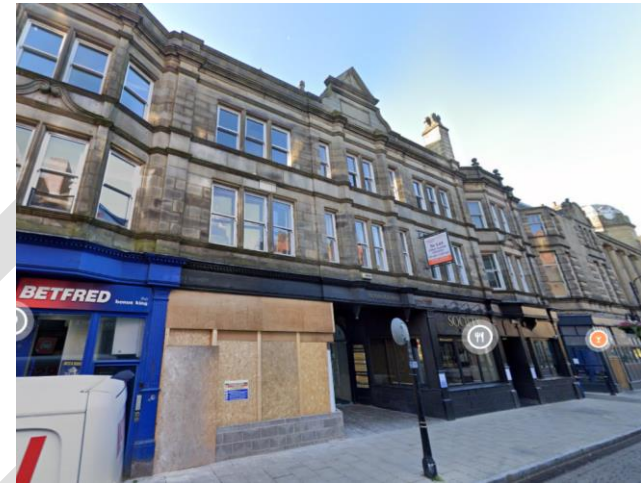
Pic 2 shows the view looking south east across Silver Street towards the western façade of Victoria Buildings, with the refurbished office (in progress) and bar on the ground floor in the centre of the picture (August 2023).
