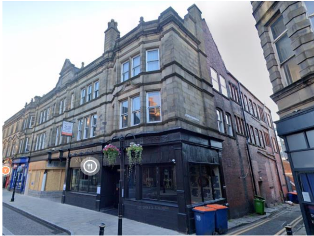
Pic 1 shows the view looking north east across Silver Street towards the western façade of Victoria Buildings, with the refurbished bar on the ground floor in the centre of the picture (August 2023).
