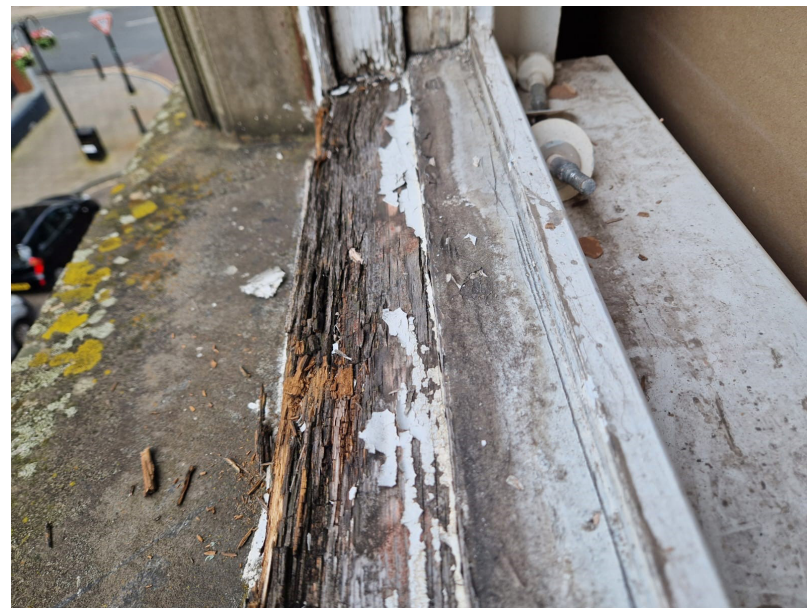
FIGURES 24 - 27 | SHOWING TYPICAL DETERIORATION OF EXISTING TIMBER SASH WINDOWS
