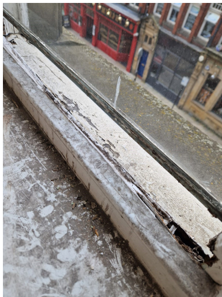
FIGURES 24 - 27 | SHOWING TYPICAL DETERIORATION OF EXISTING TIMBER SASH WINDOWS
