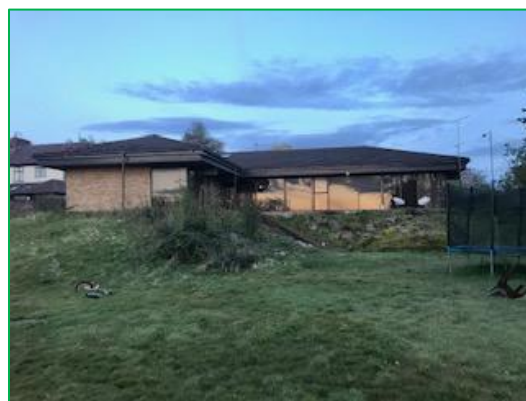
The northwest elevation of the building
