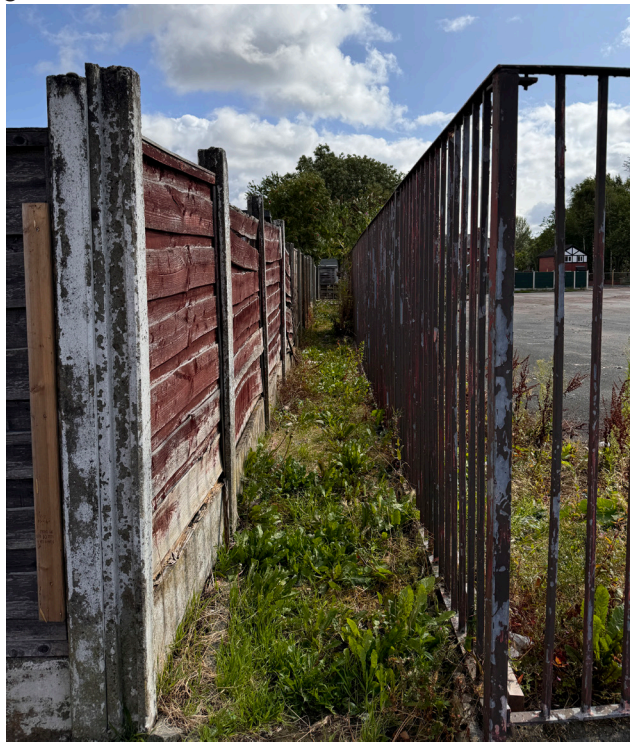
⑩ View within site towards western boundary. Existing walls to be retained with new 2.4m high paladin fence set behind.
