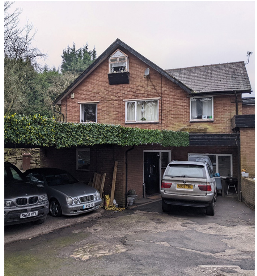
Figure 1: View towards existing dwelling from the east of the site
