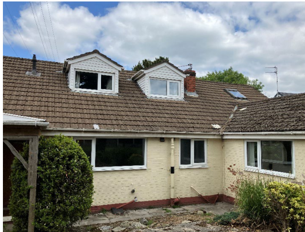
Photo 2: 15 Radcliffe Moor Road Rear Elevation
