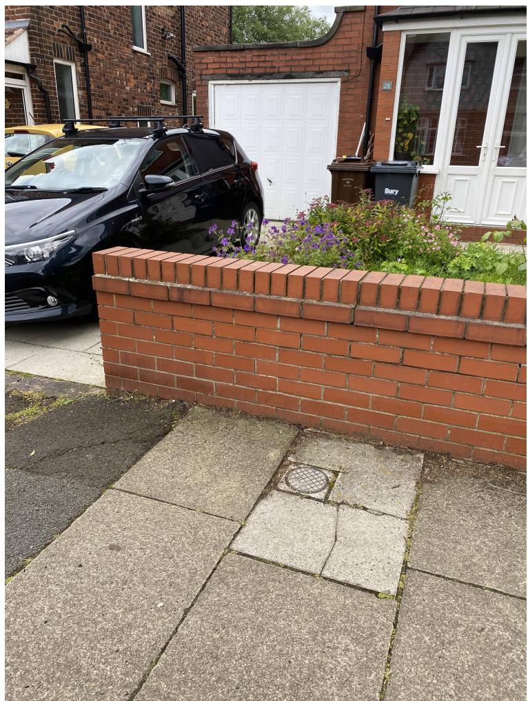
Front boundary wall Stack bond head with protruding running bond below
