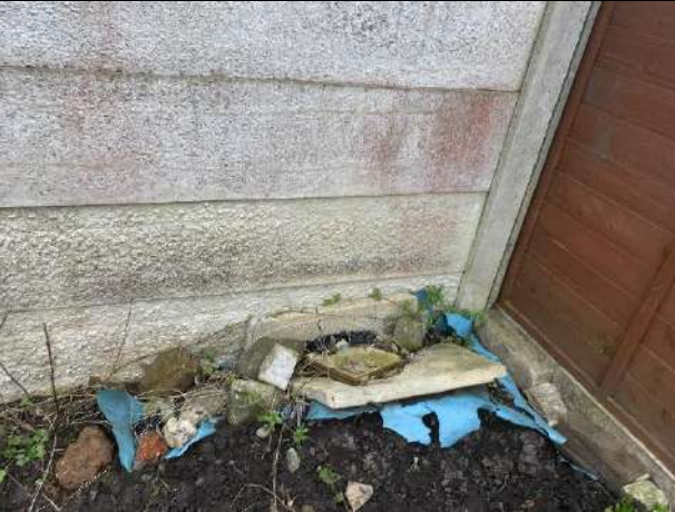
P5: Small stockpile of hardstanding material in the northern corner of the site.
