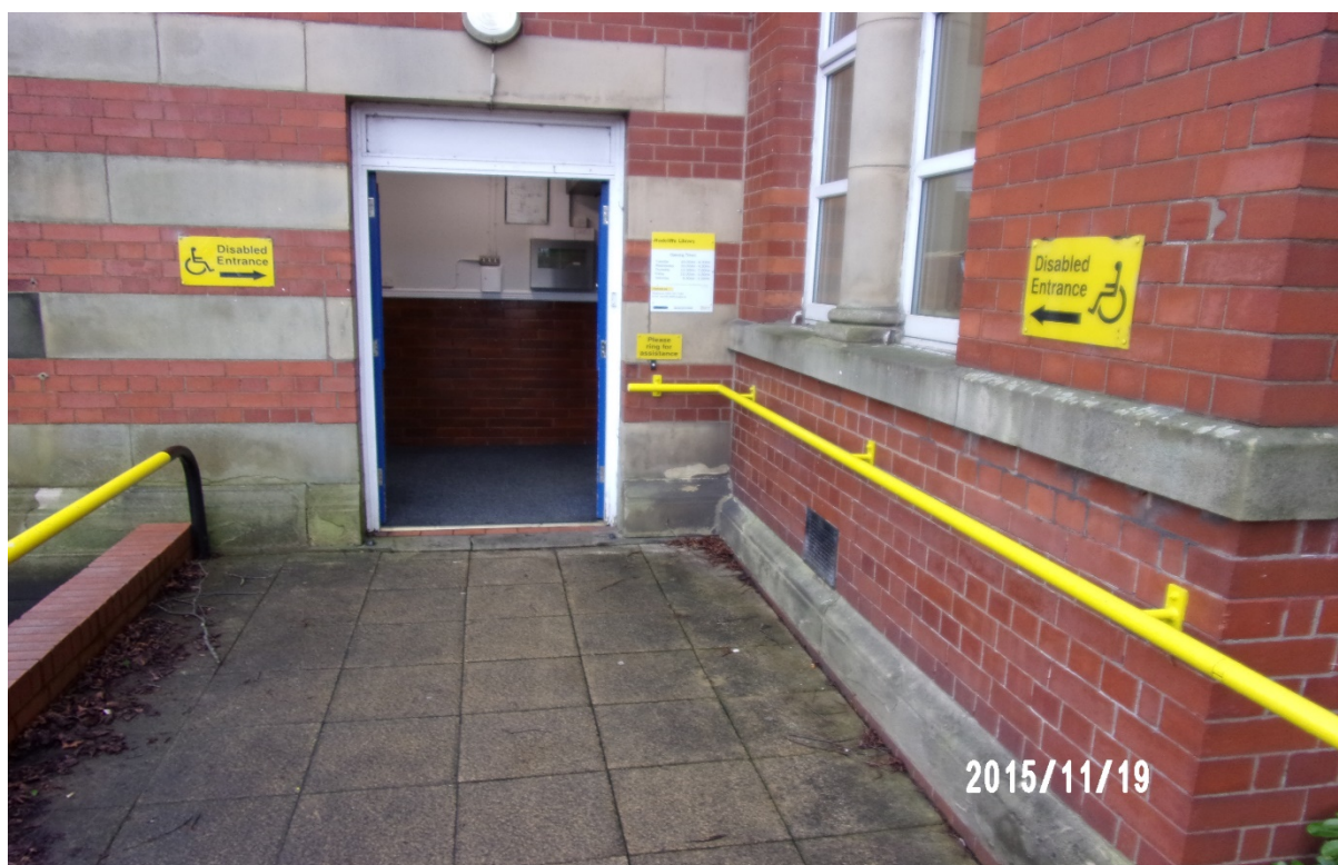
PHOTO 10 : Showing smaller replacement signage to the side ramp entrance.
