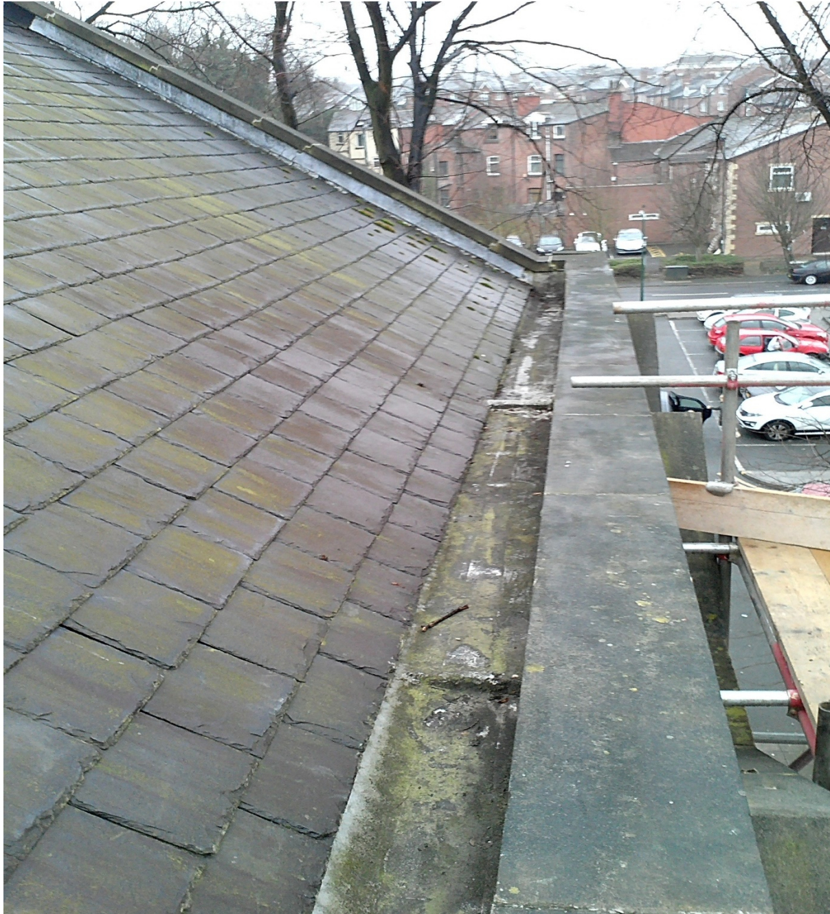
PHOTO 1 : FRONT ELEVATION – Showing Pitched roof and low brick with stone coping parapet detail & lead lined flashing that steps down towards each end to wall outlets. It is proposed to replace in a felt detail taken up the wall ( like photo 2) to form a better seal and out onto the top of the coping.
