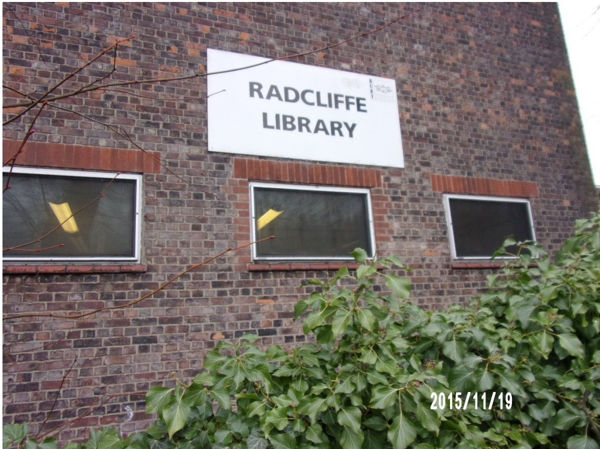
PHOTO 12 : Showing the only original sign ( old corporate logo ) still in place to the car park gable elevation wall.
