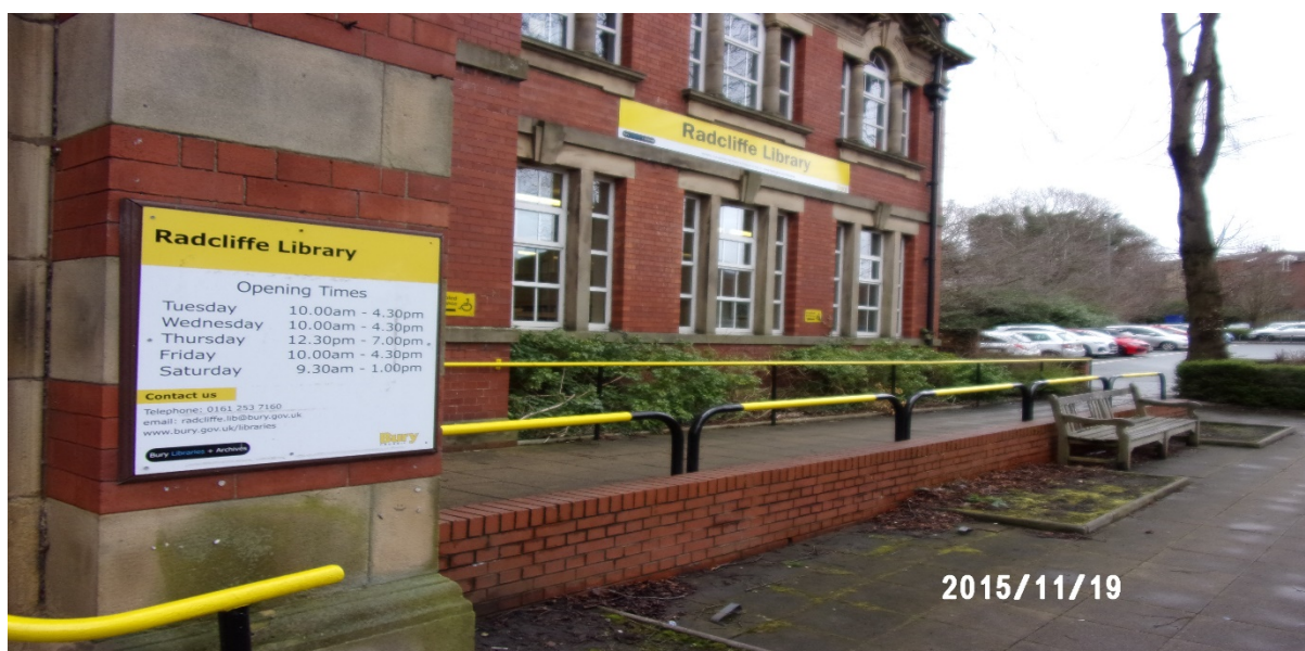
PHOTO 11: Showing front elevation view from the front door & library opening times sign
