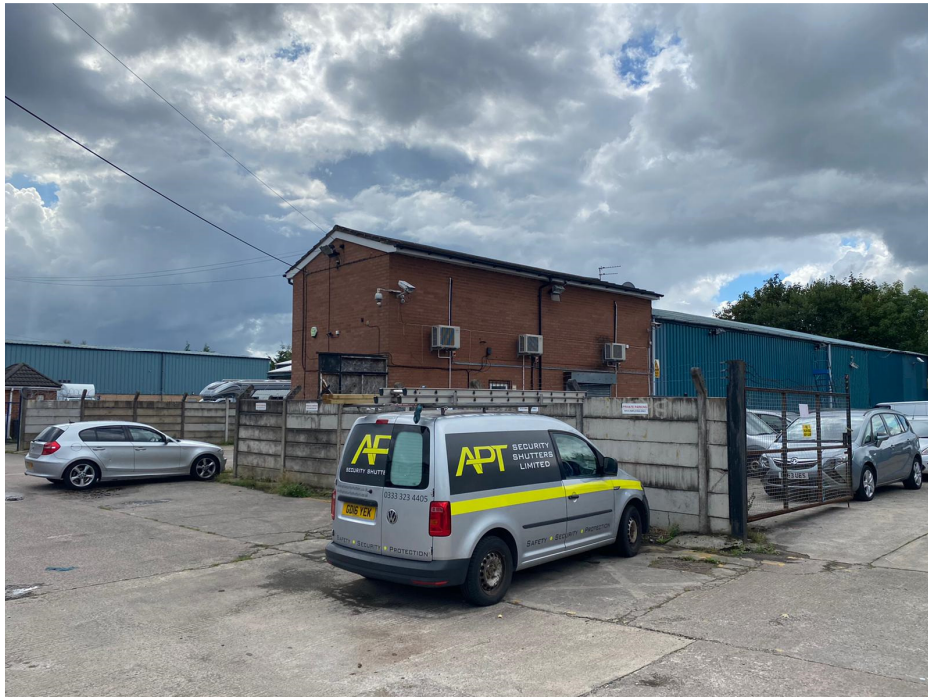
Photo of plot main entrance illustrating the maximum 1:48 approx fall across the site meaning a fall of around 340mm from the front of the plot to the rear of the plot (location of the units).
