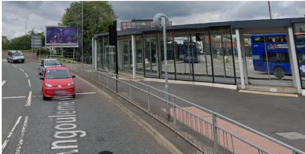
Large advertisement hoarding adjacent (west) of the application site
