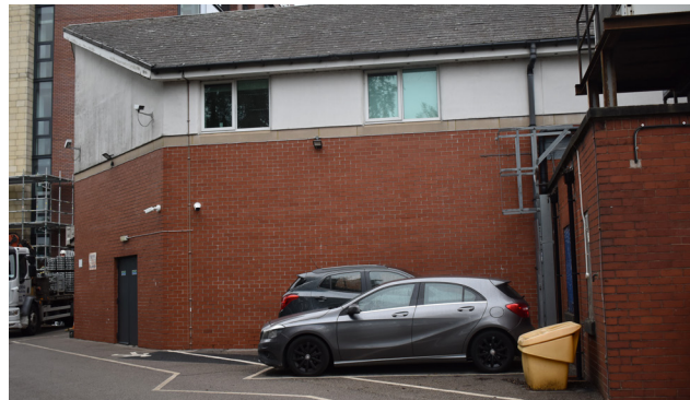
3.56 Modern rear range (Catering Wing), south and west elevations
