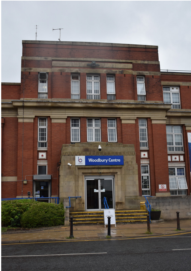
3.42 East Wing, east elevation, south entrance portico
