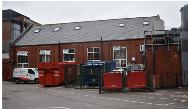
3.53 Former Gymnasium, south elevation
