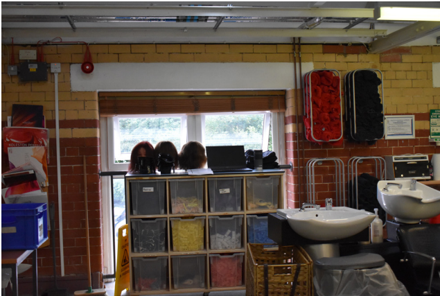
3.81 Former Gymnasium, historic brickwork
