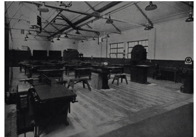
2.26 Carpentry and Joinery Workshop, 1947 (Bury Archives)
