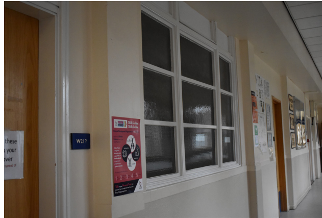
3.72 Room 212, Window to corridor
