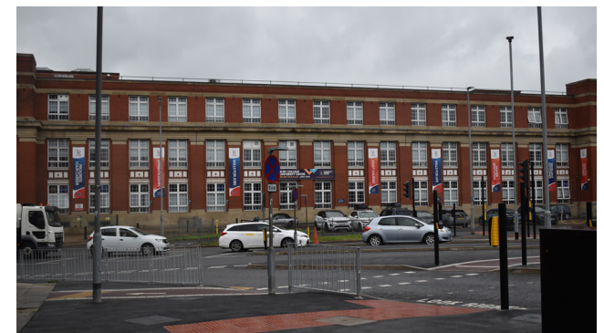
3.39 East Wing, east elevation, main range
