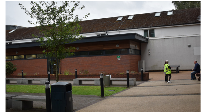
3.58 Modern rear ranges (Catering Wing), north elevations
