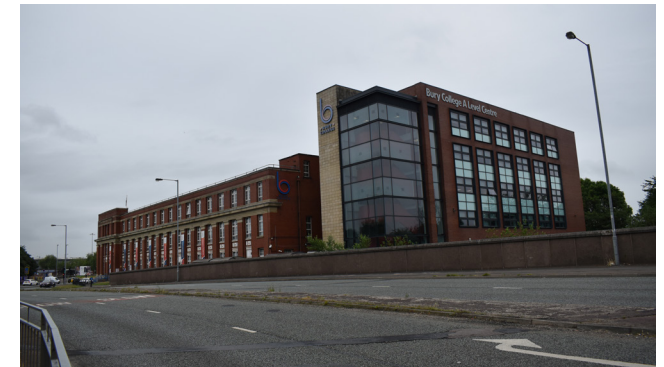
3.19 A Level Centre, west elevation
