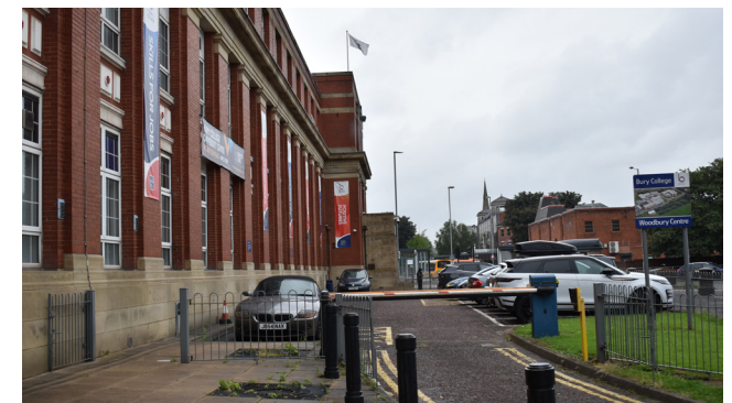
3.25 East car park and access road
