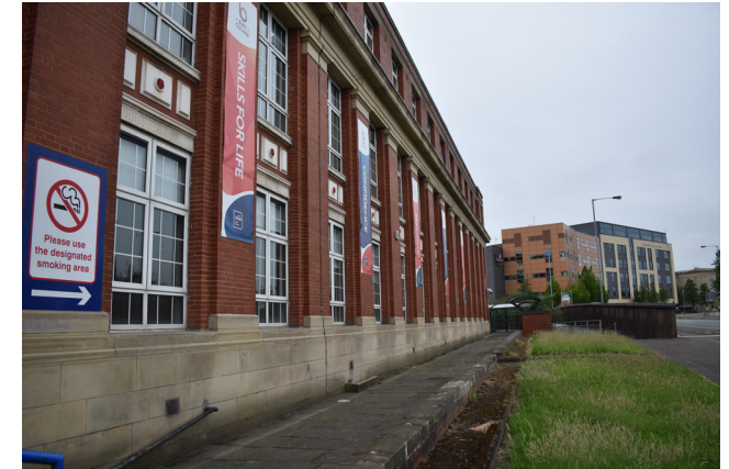
3.20 North elevation, former walled pathway
