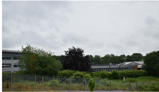
3.13 South campus, north perimeter, viewed from Market Street
