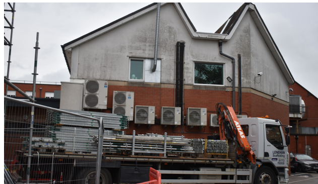
3.57 Modern rear range (Catering Wing), west elevation
