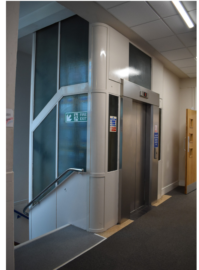
3.77 North entrance lift
