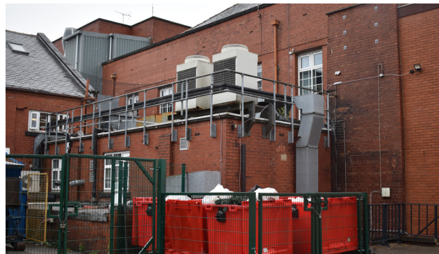
3.52 East Wing, rear (west), single-storey structure
