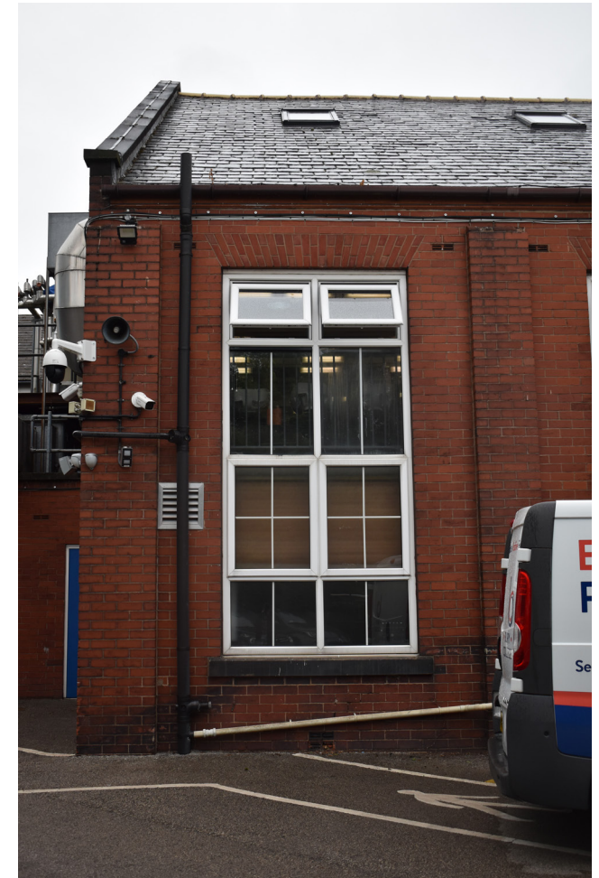
3.54 Former Gymnasium, south elevation, example bay
