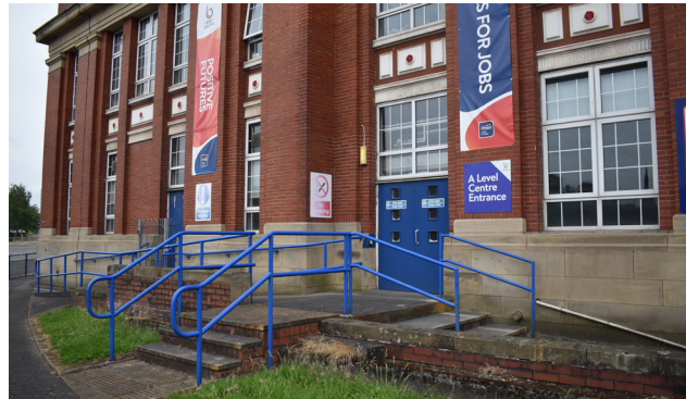
3.21 North elevation, inserted entrances with modern ramps, steps and railings, and truncated footpath and wall
