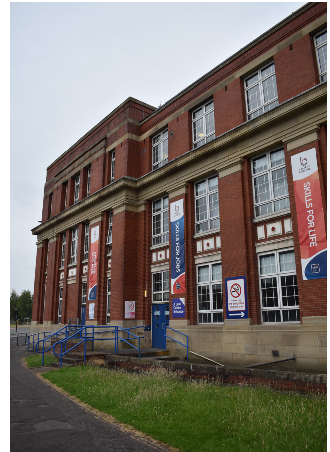
3.49 North elevation, projecting north pavilion
