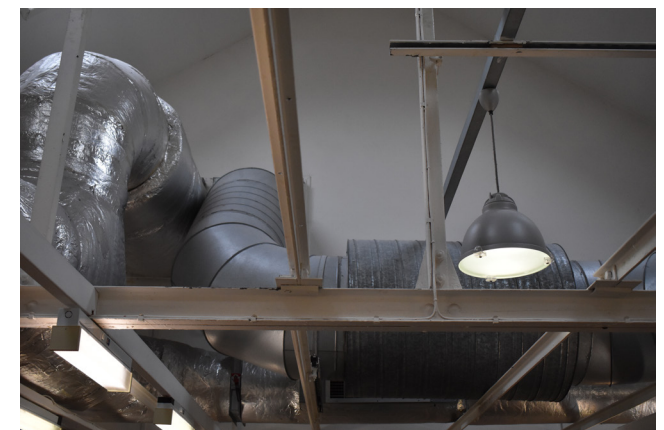
3.80 Former Gymnasium, ducting
