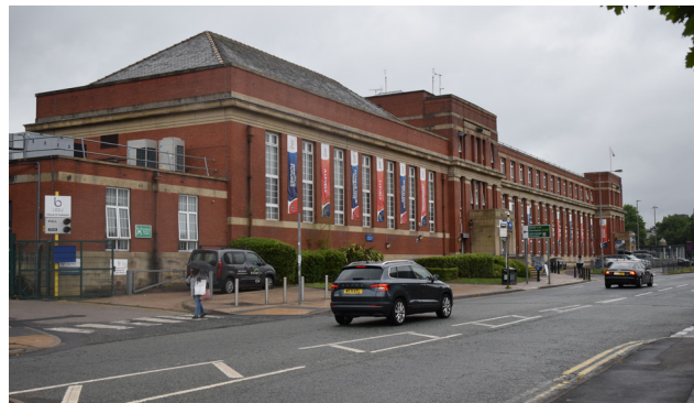
3.45 East Wing, east elevation (with North Wing, east elevation to the north)
