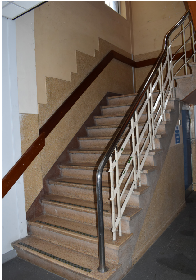
3.76 West exit stairs
