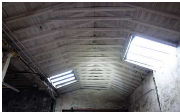
Timber clad roof area.
