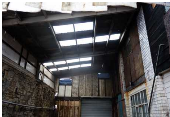
Single skin roof with no roost features
