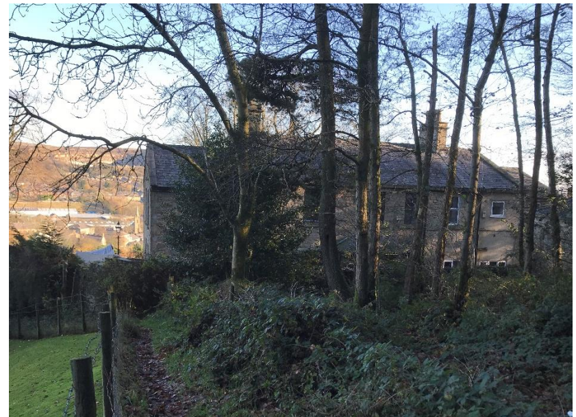
Figure 4.16: The rear elevation of Prospect House
