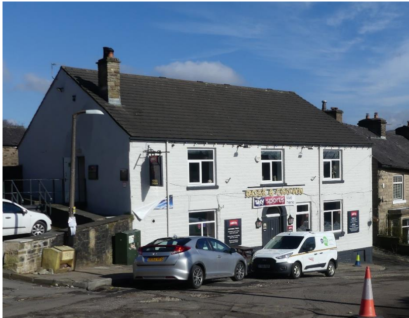
Figure 4.18: The front elevation of the Rose and Crown Public House
