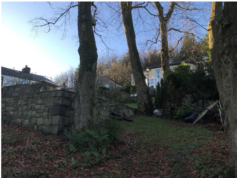
Figure 4.17: The retaining wall to the southern garden
