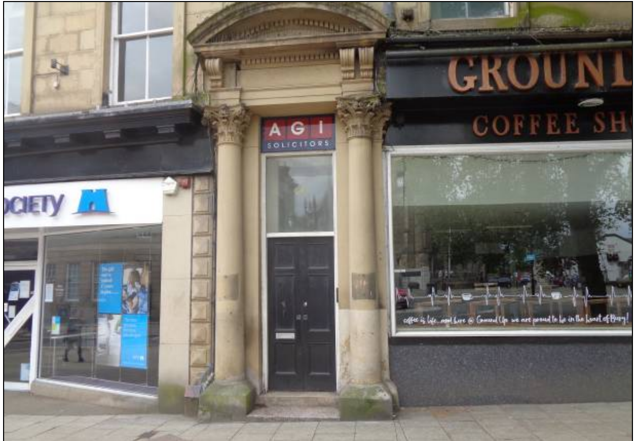
4. Tall pedimented entrance to the offices on the upper floors
