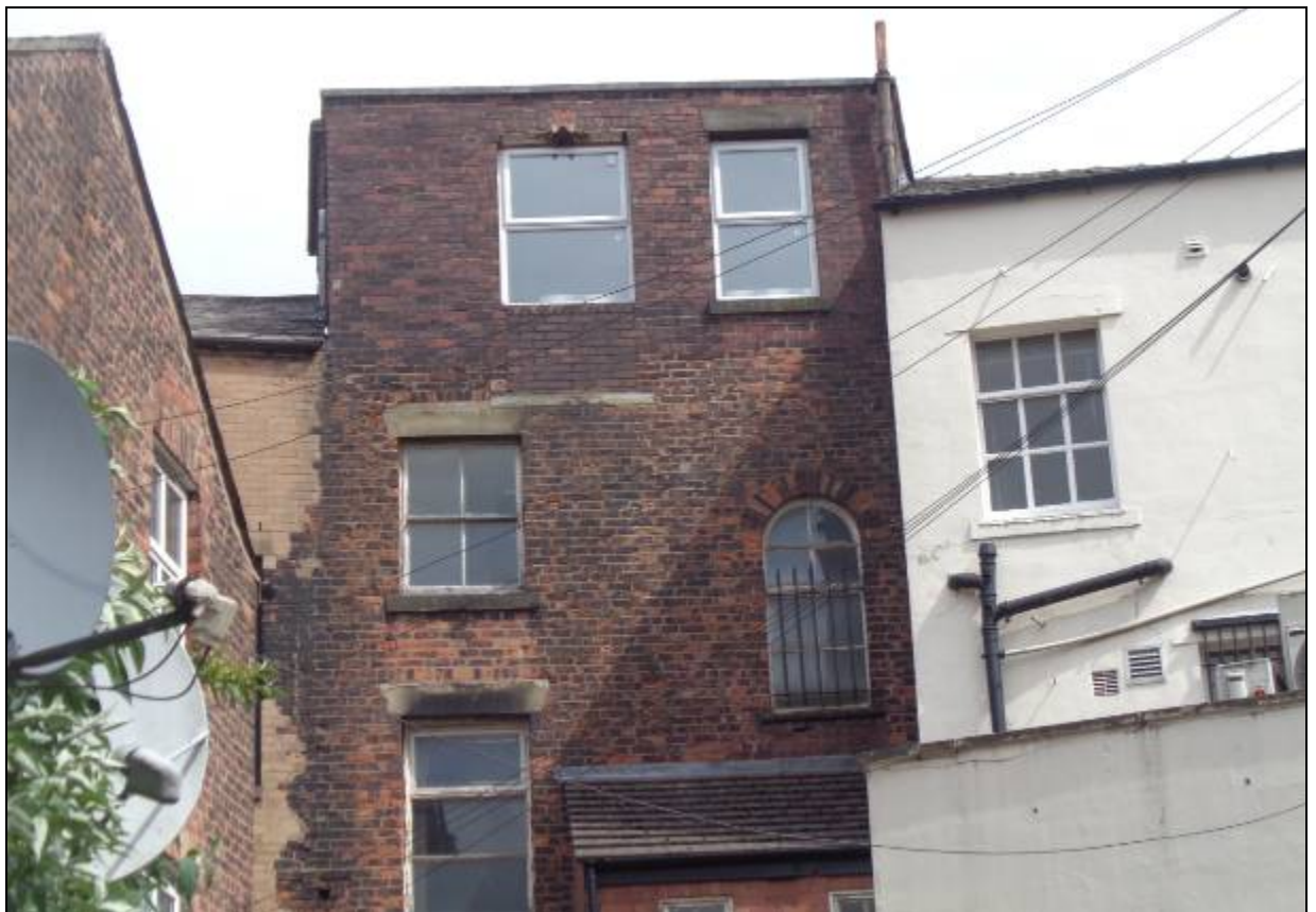
6. Rear elevation has a more irregular, workaday appearance
