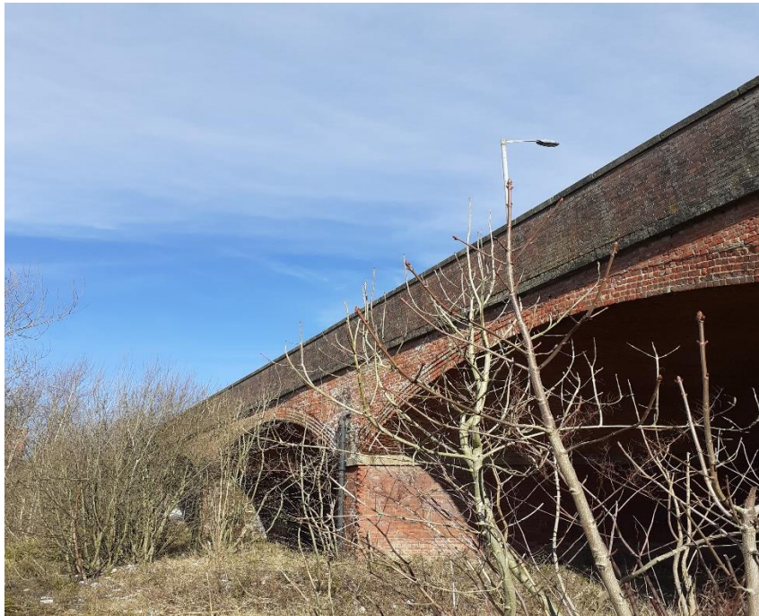
Figure 5: Market Street Arches
