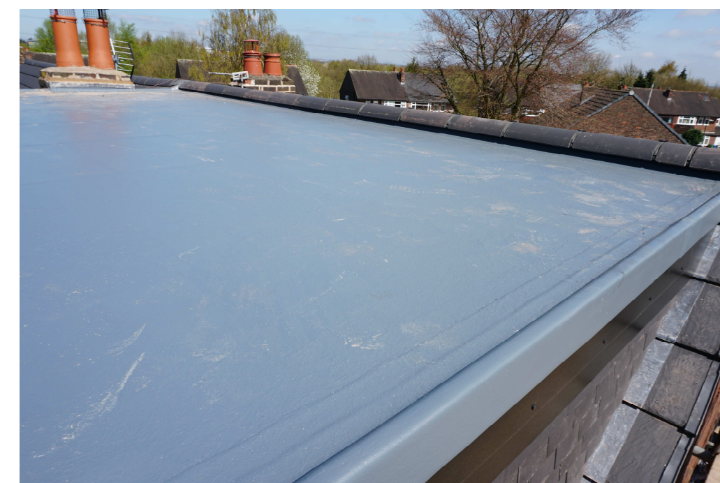
Typical Fibreglass Finish to New Flat Roof
