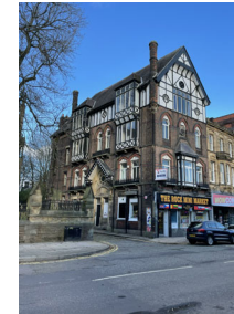
Street view showing facade
