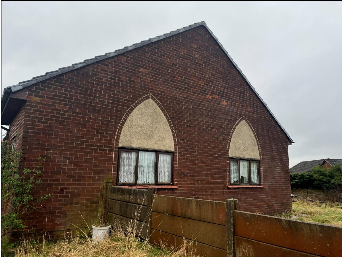
Plate 17 – Eastern aspect of the building, with tight gapping and verges noted
