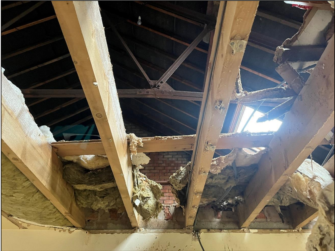
Plate 19 – Character of the loft space as seen from ground floor, with roof lining and skylights
