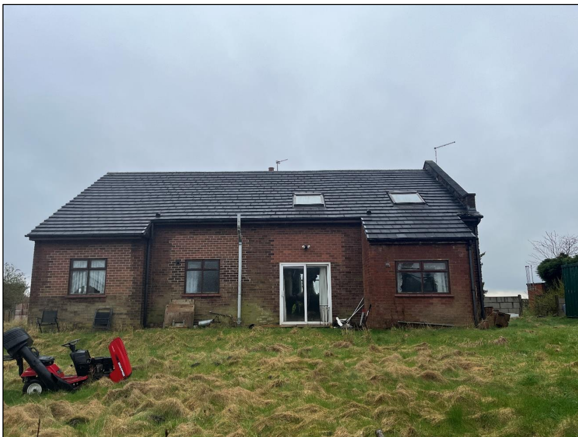
Plate 7 – Rear aspect of the dwelling
