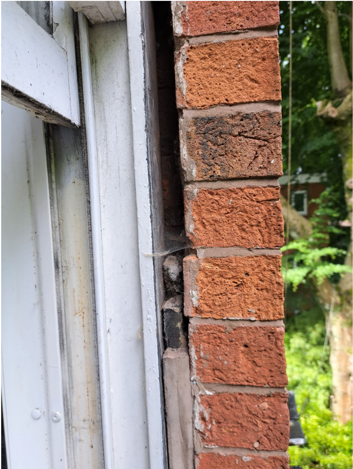
Upstairs Window Reveal:
