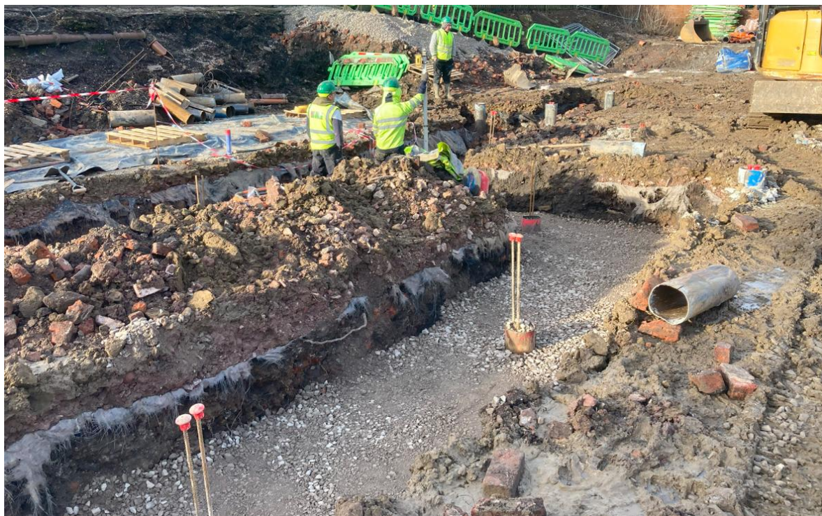
PLATE 2 EXCAVATION OF TRENCHES FOR BUILDING FOUNDATIONS
