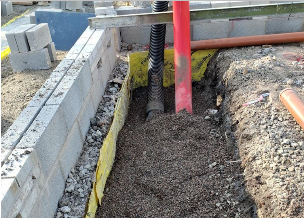
FIGURE 4.1 INSTALLED BARRIER (TYPE A) PIPEWORK
