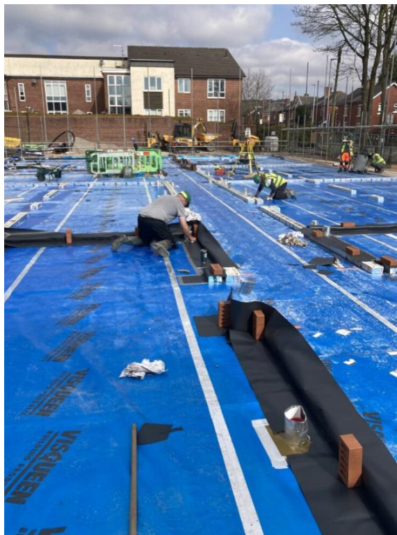
PLATE 4 INSTALLATION OF VAPOR GAS MEMBRANE
