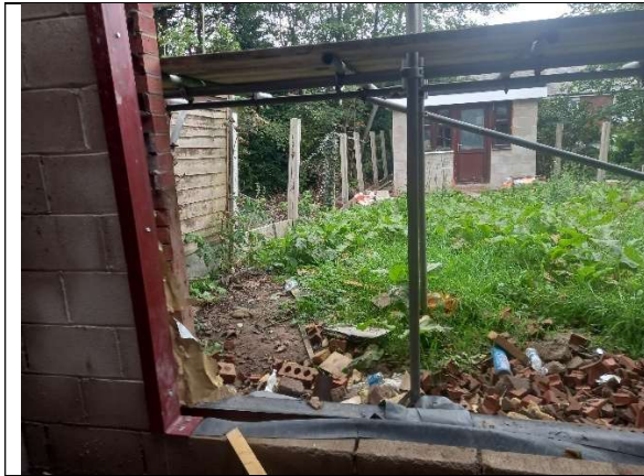
Photograph 3: View of rear garden. Note shed on concrete base.
