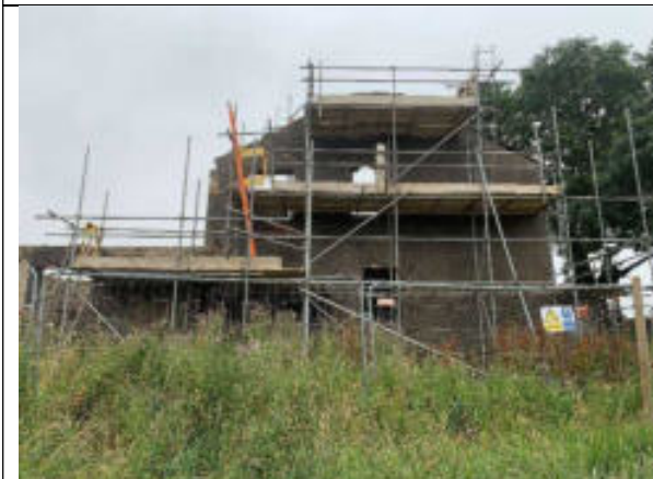
Photograph 3: Existing building on site- taken facing north.
