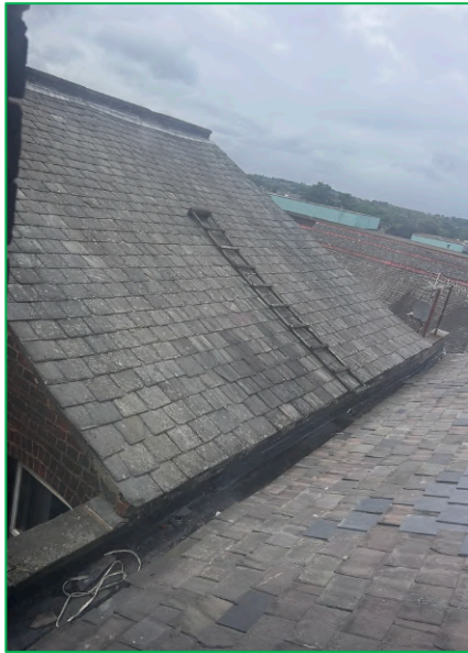
Showing the well-fitted slates on the north elevation of the western end of the building
