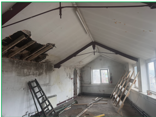
Showing the sealed upper floor
