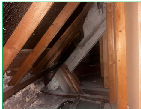
Showing the accessible eaves in the attic space
