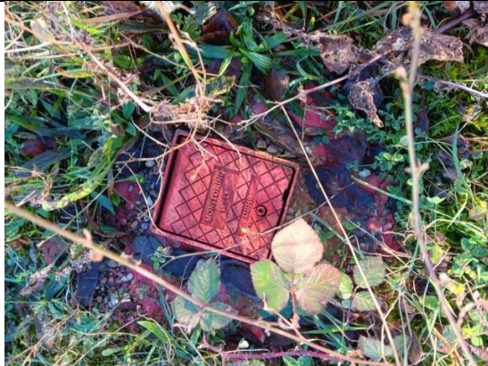
Photograph 5: Existing groundwater monitoring well.
