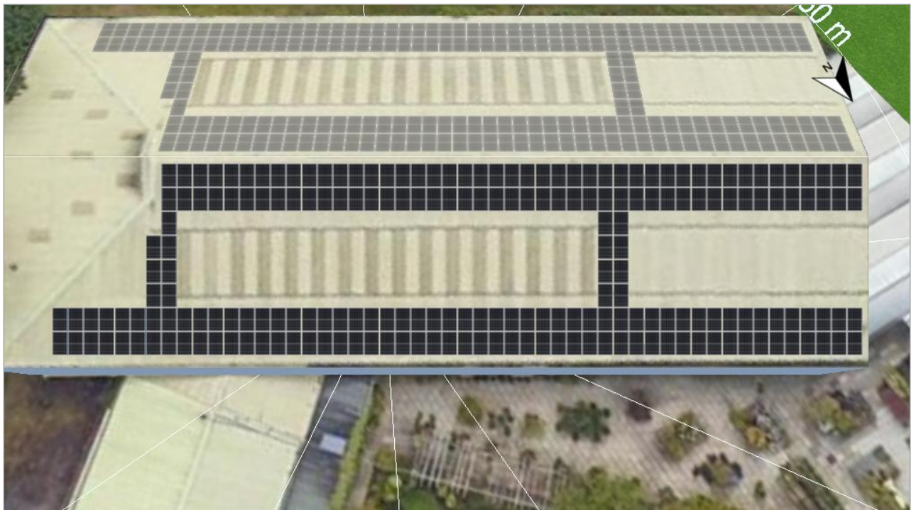
Figure: 2. Module Area - Building 01-Roof Area Northeast
