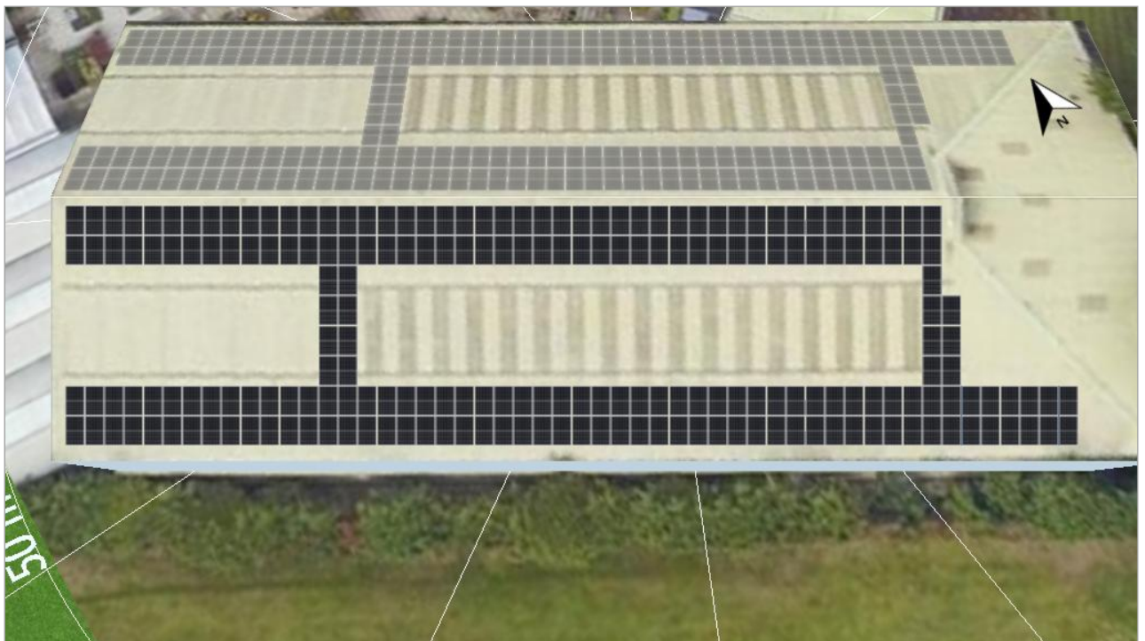
Figure: 1. Module Area - Building 01-Roof Area Southwest
