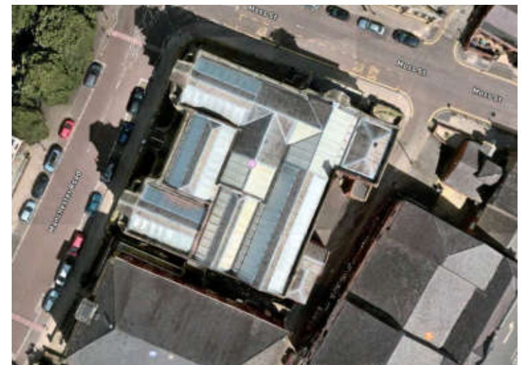
04 Aerial view of roof, orientated to North (c) Google.
