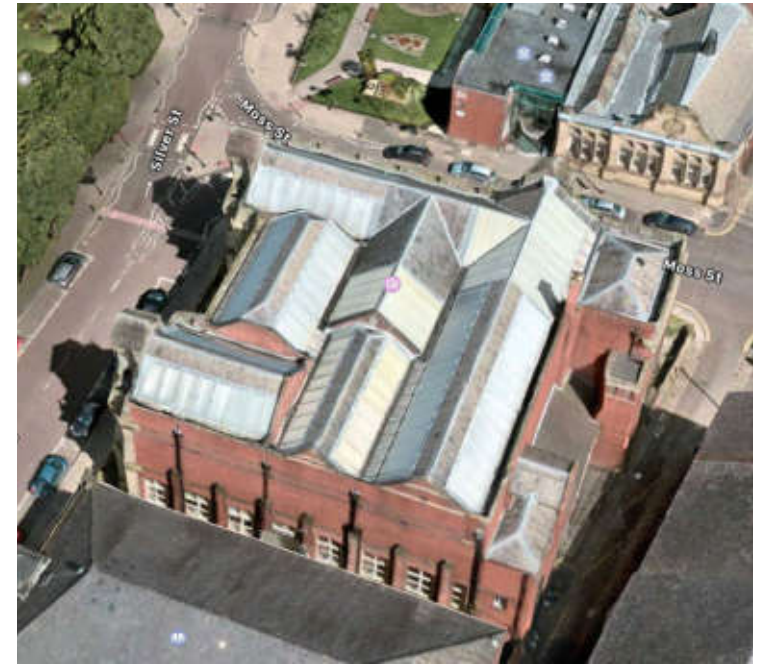
03 Oblique (aerial) view of roof, looking North. (c) Google.
