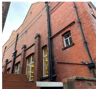
11 General view from Back Knowsley Street (2023)
