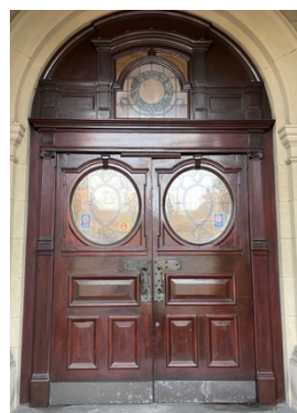
14 DG01 fine entrance doors with fanlight (2023)
