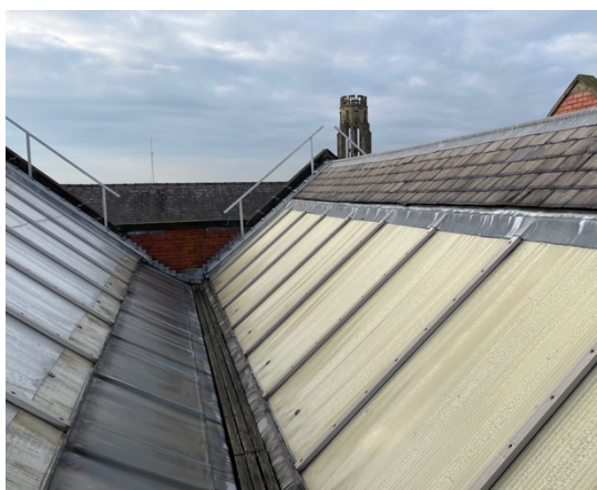
03 Polycarbonate rooflights in Area 07 (2023)
