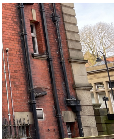
07 Configuration of RWP02 which drains Roof Area 1 (2023)
