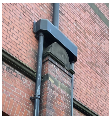
08 RWP09 hopper and split above buttress (2023)
