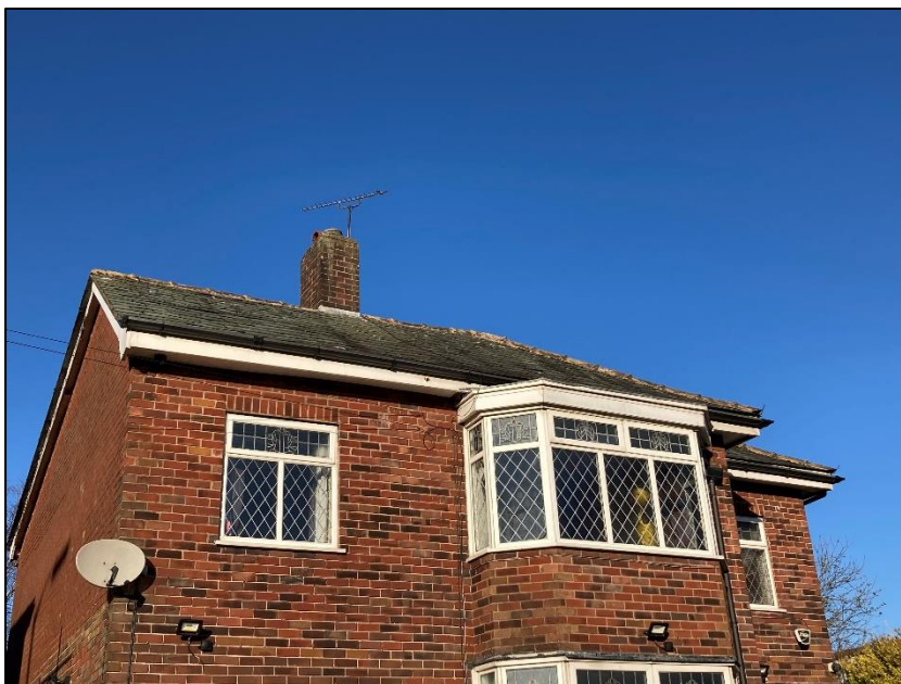
Photograph 3 showing the roof at the front of the property
