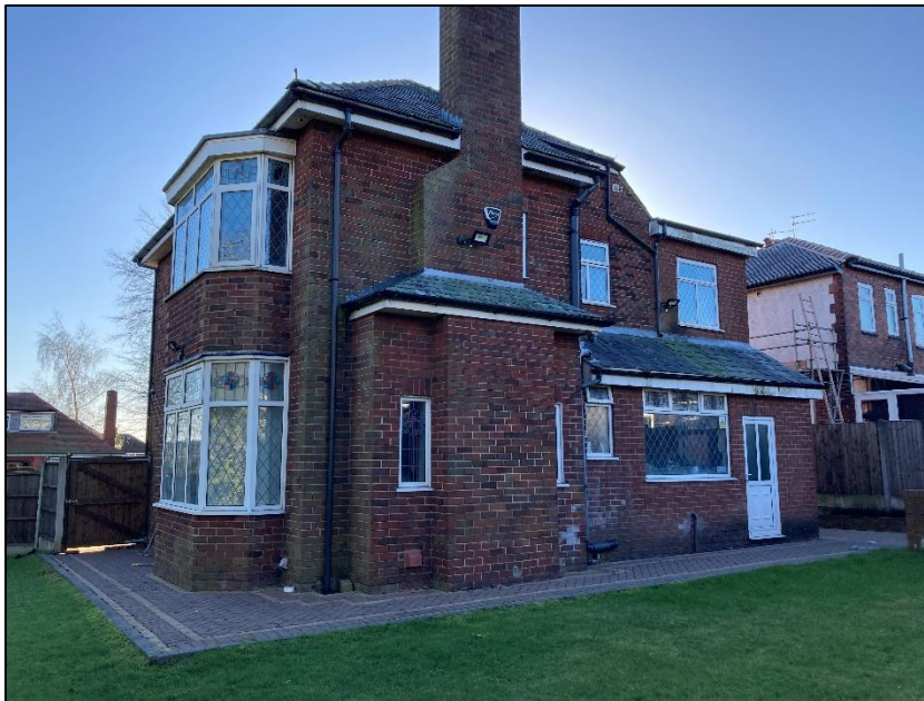
Photograph 1 showing the rear of the building
