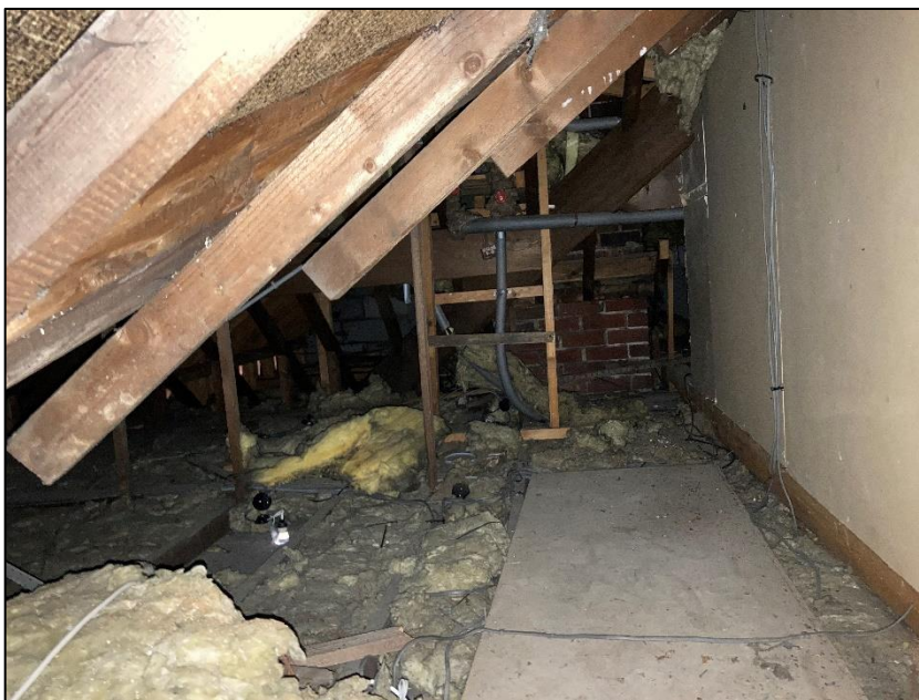
Photograph 7 showing the space under the eaves
