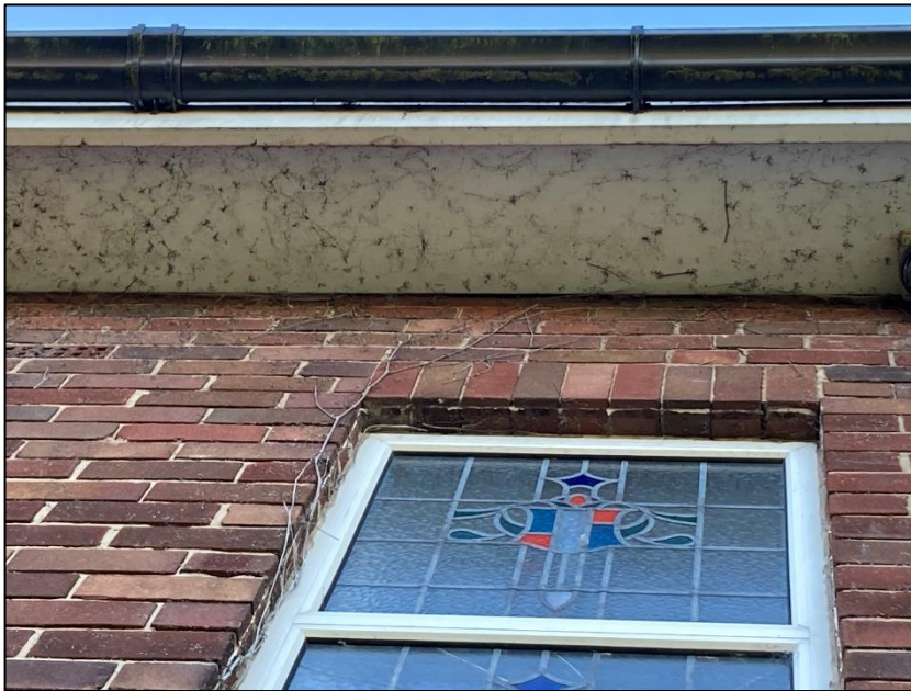
Photograph 4 showing the uPVC soffit and bargeboards
