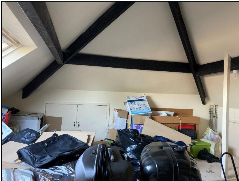
Photograph 6 showing the section of roof void used for storage
