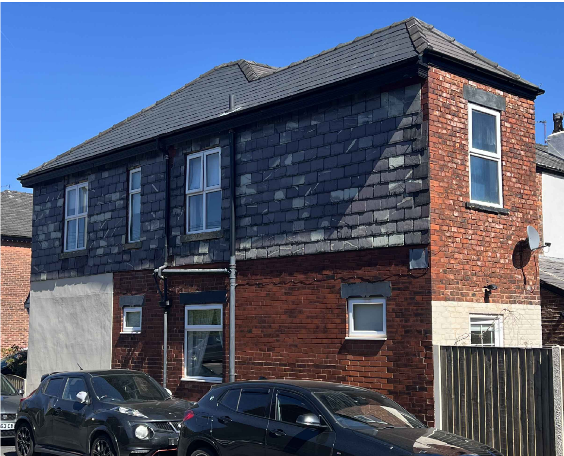
Existing Side/Rear Elevation
