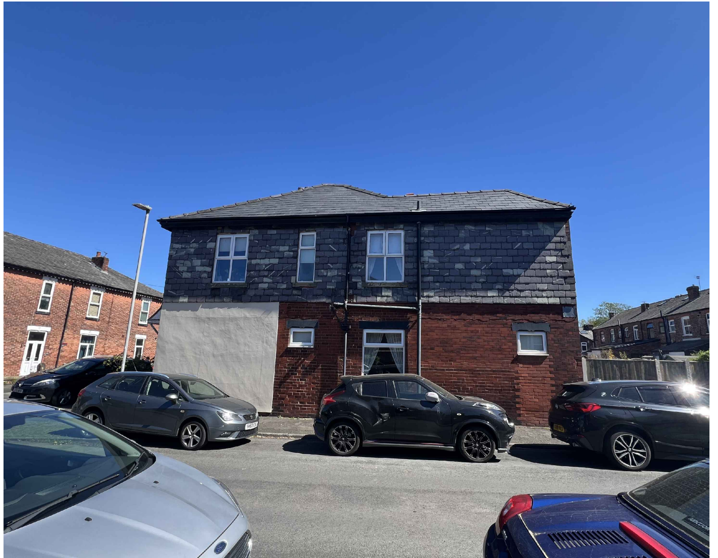
Side Elevation of Site
