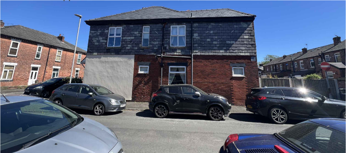
Side Elevation of Site
