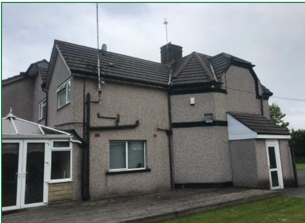
The south elevation of the house
