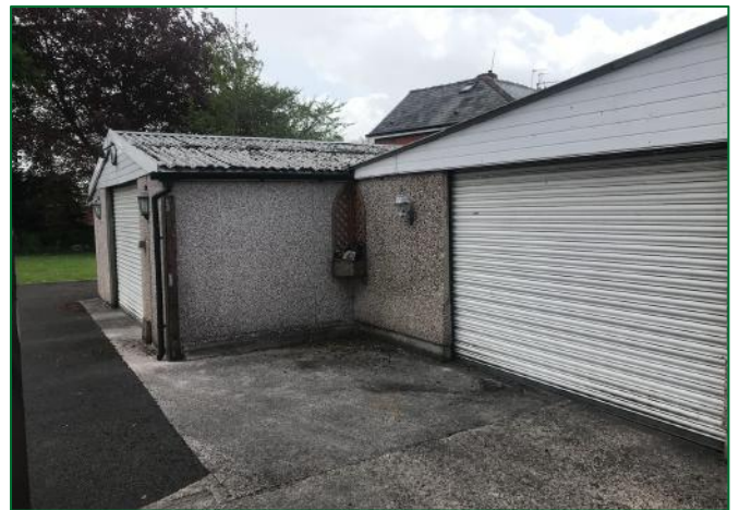
The north and west elevation of the garage
