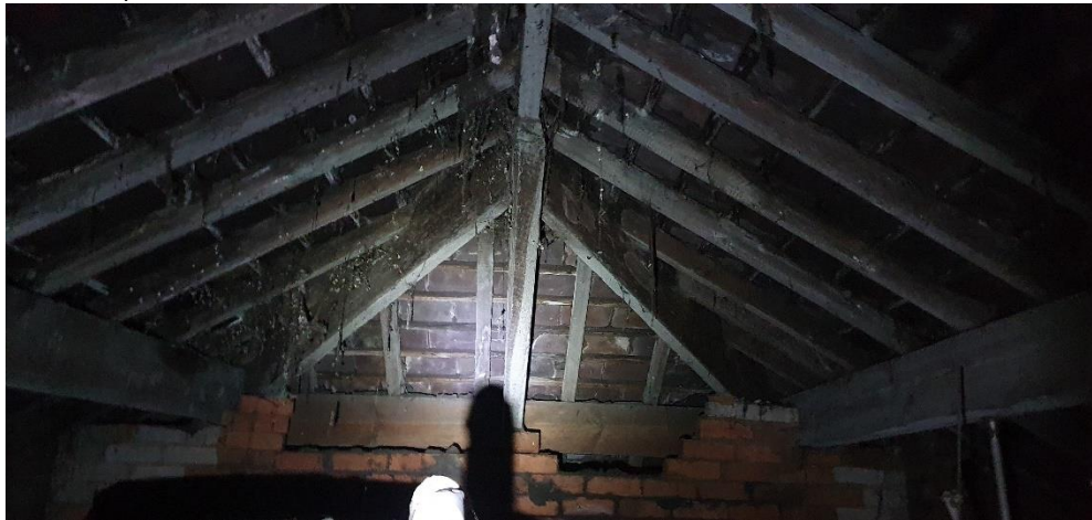
B1 - loft interior looking east
