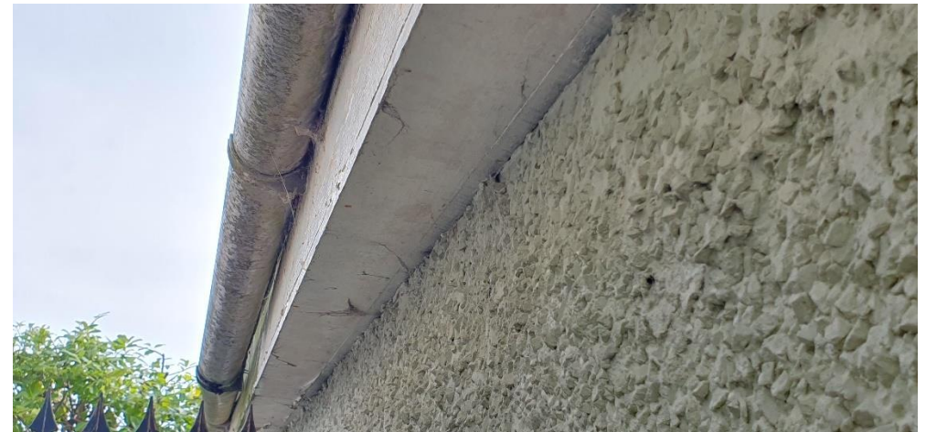
B1 – well sealed soffits
