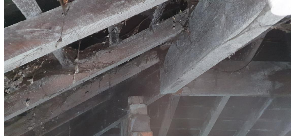
B1 - example of underside of the roof tiles
