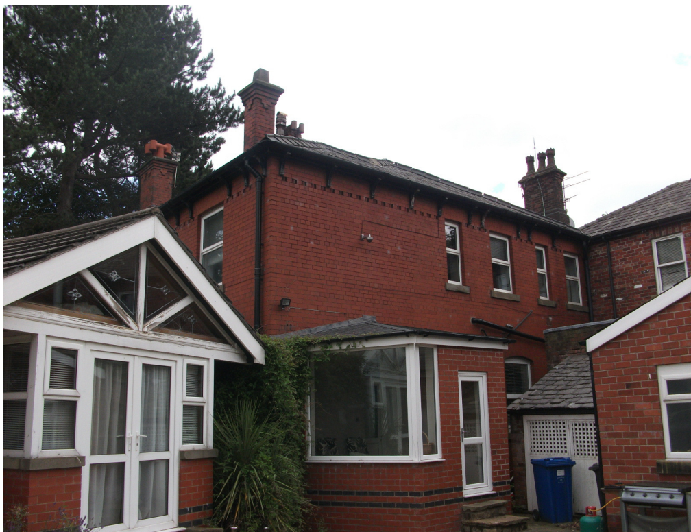
REAR WALL OF ORIGINAL PROPERTY
