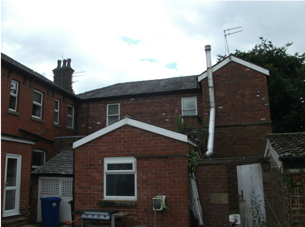
RIGHT HAND WALL OF MAIN EXTENSION AND SINGLE STOREY EXTENSION
