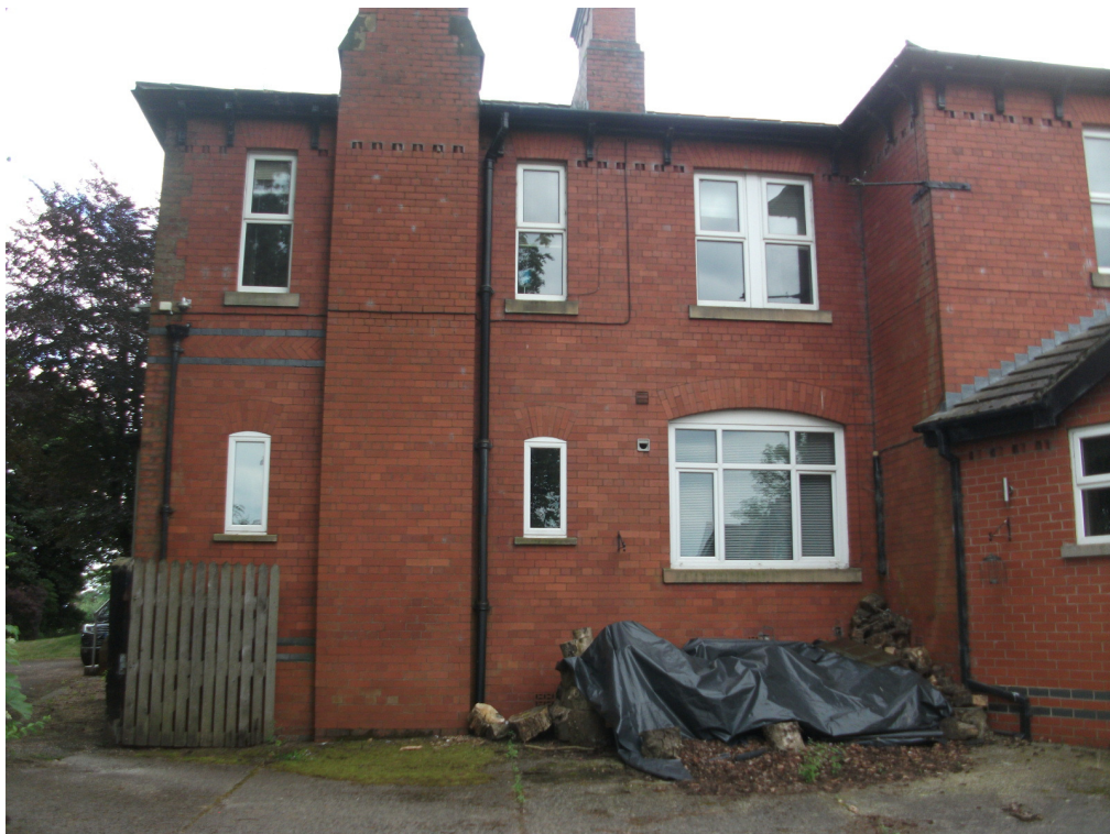
RIGHT HAND WALL OF ORIGINAL HOUSE
