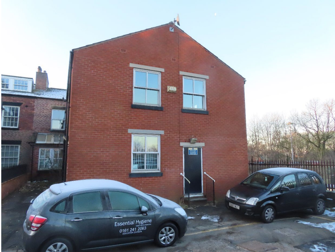
Two storey extension to outrigger of number 18/20.
