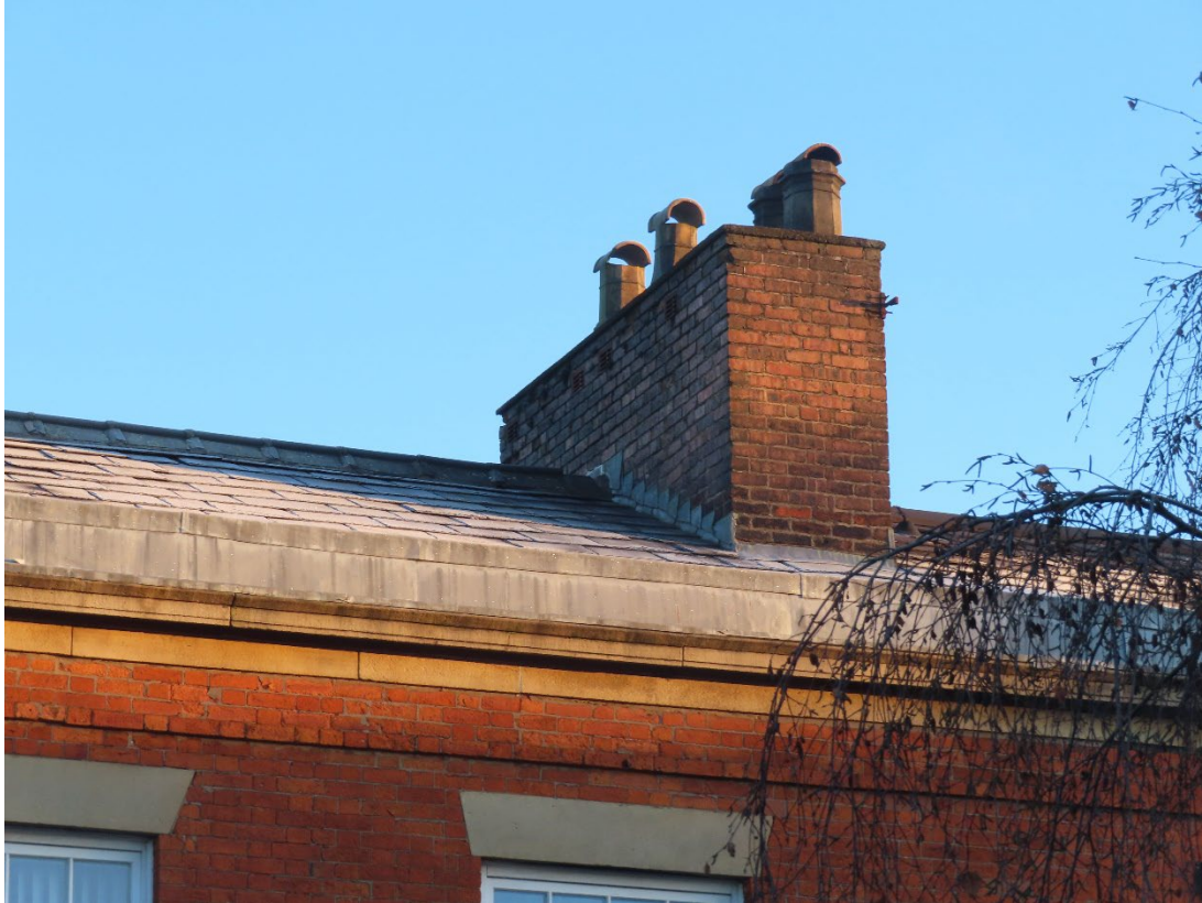
Re-pointing of chimney stack to number 18.
