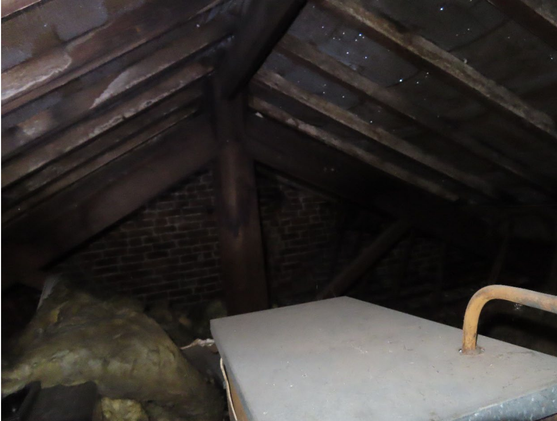
King post truss to roof of outrigger to number 18/20.
