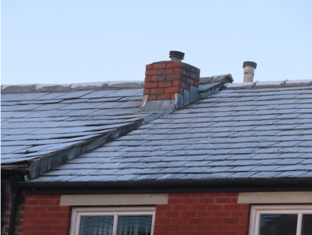
Repair single stack to outrigger of number 18.
