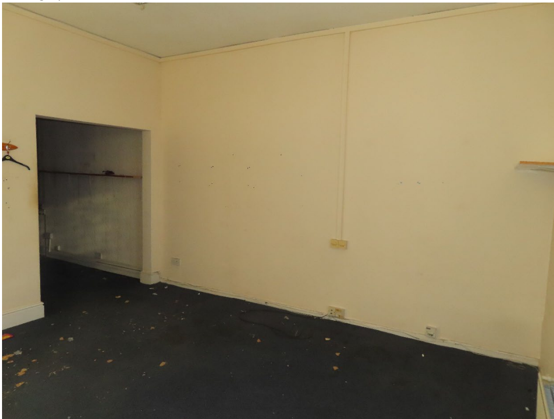
Chimney breast removed to reception office to number 18 (means of support?).
