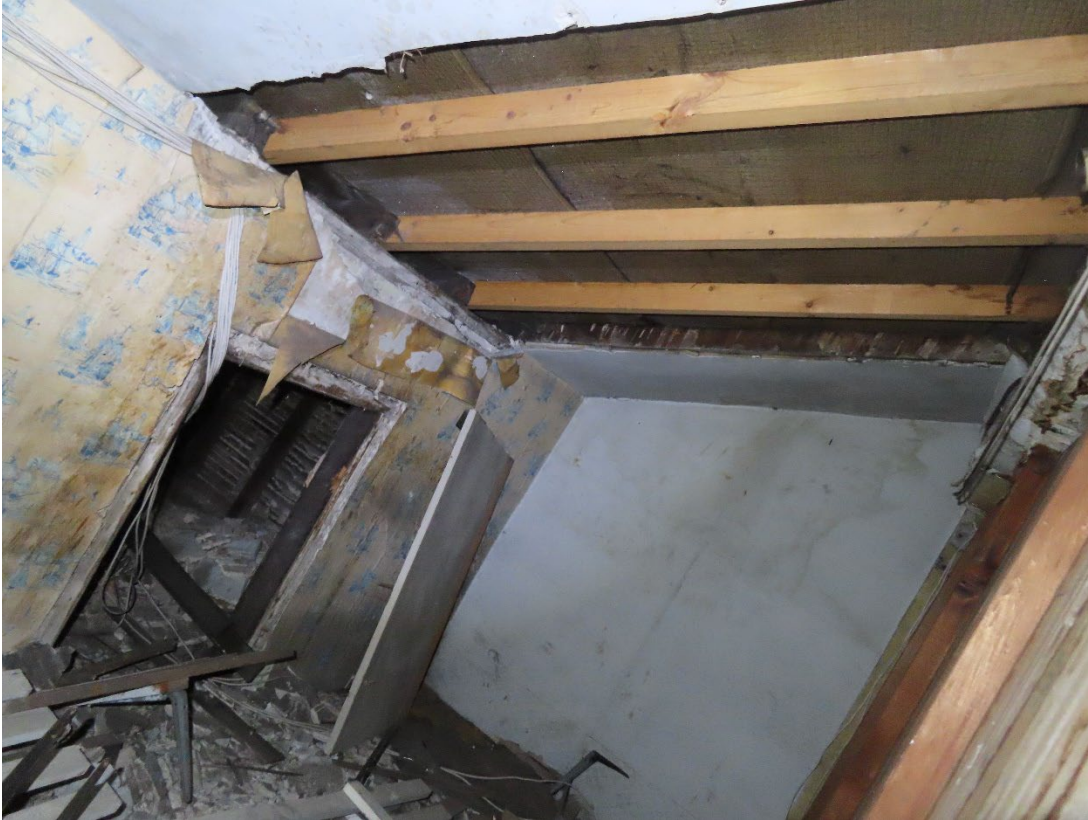
Section of rafters replaced to main roof of number 20.
