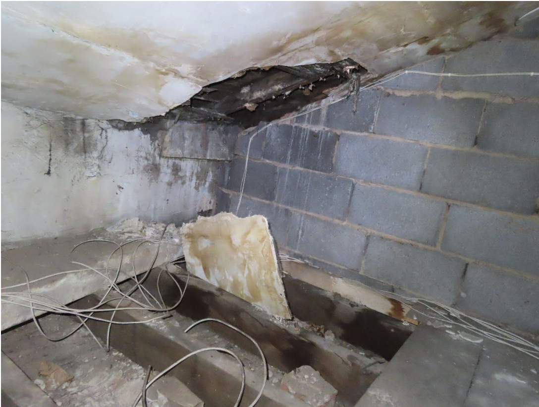
Rear roof of number 20 showing over boarding and rebuilt gable and rear wall.
