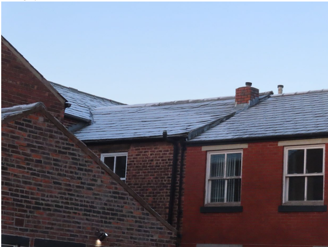
Clipped slate to main rear roof and original outrigger to number 18.
