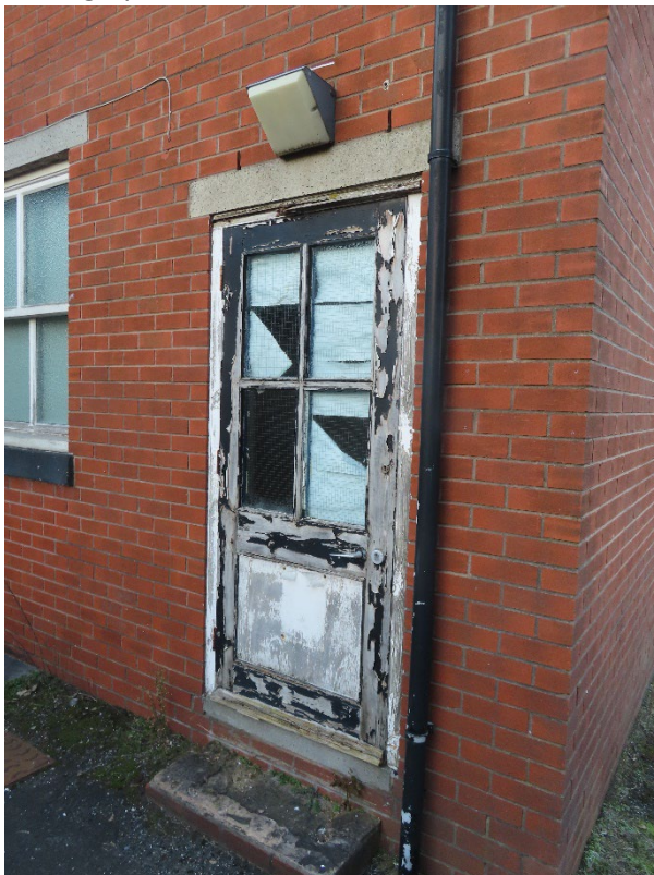
Localised repairs to side door of extension to number 18.
