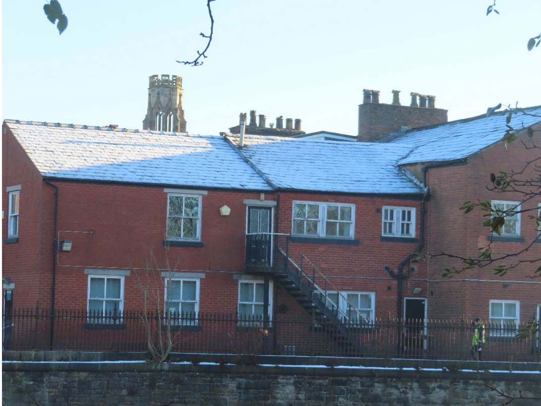
Roof of rebuilt outrigger extension to number 20 front roof covering.
