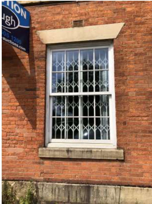
Image 5 – View of window to front elevation (No 20)
