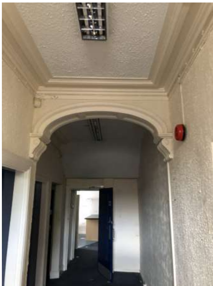
Image 16 – Internal hallway with cornice and arch detail
