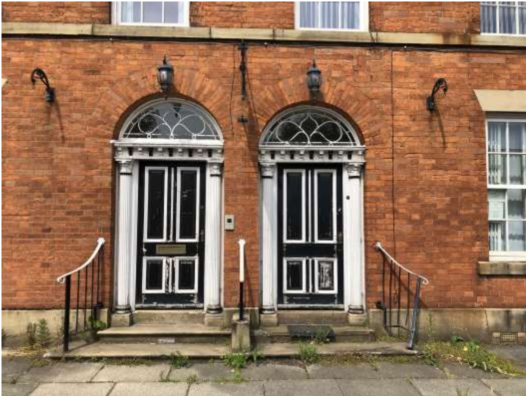
Image 3 – View of front entrance doors
