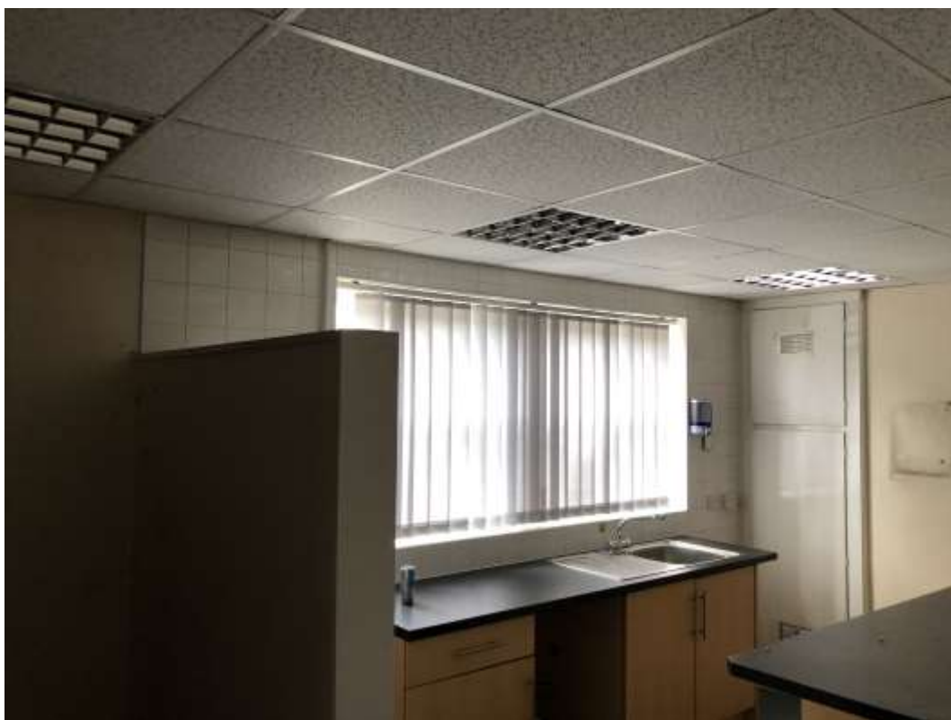
Image 19 – suspended ceiling installed in ground floor kitchen (No. 20)
