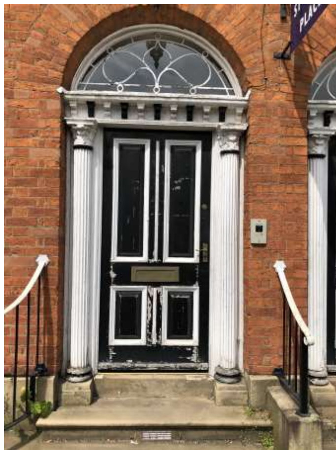
Image 4 – View of front entrance door (No 20)
