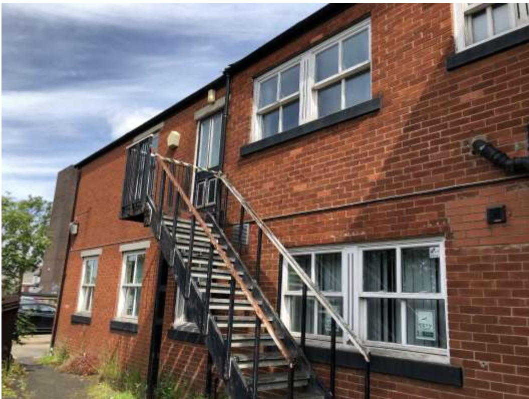
Image 8 – Side elevation (west) and external fire escape/stairs
