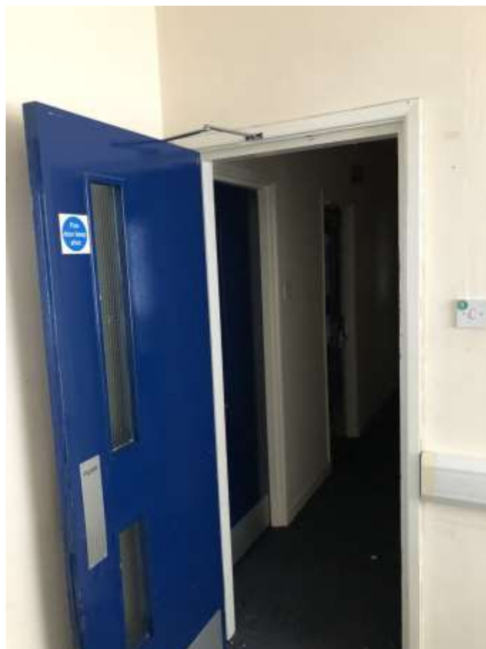
Image 20 – Modern internal door & architrave
