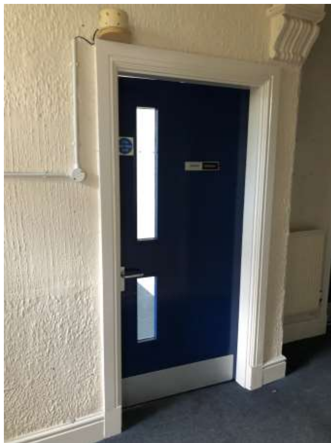
Image 18 – View of internal door and architraves within hallway
