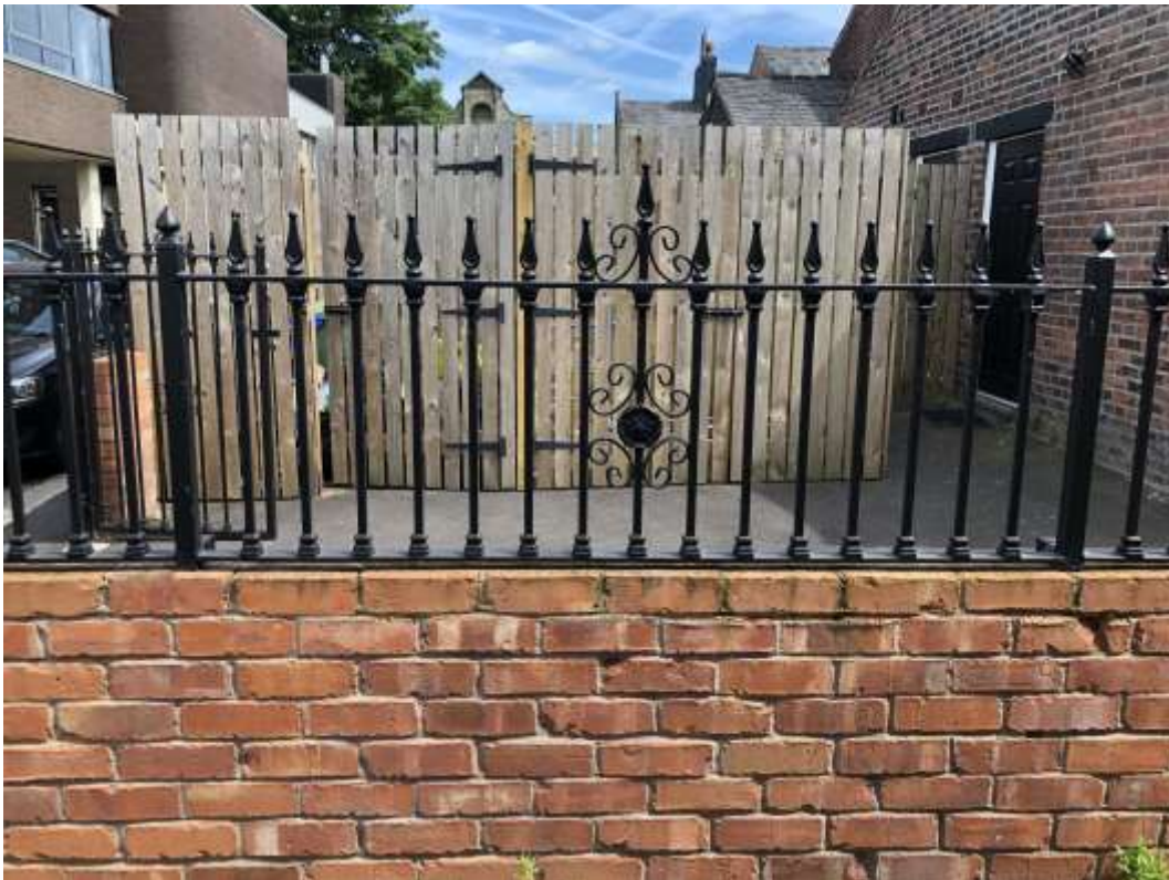
Image 14 – Brick wall and railing forming boundary division at rear
