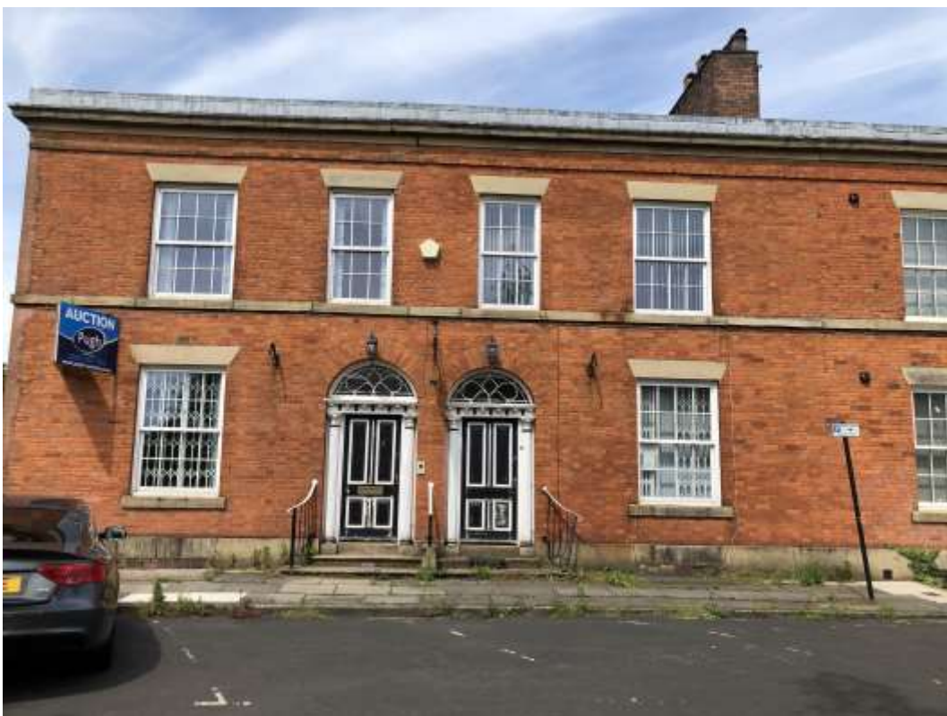
Image 2 – View of front elevation
