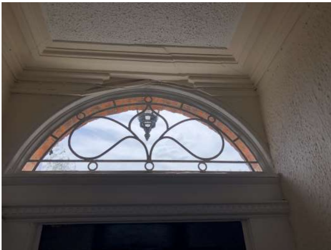
Image 15 – Fanlight to front entrance door
