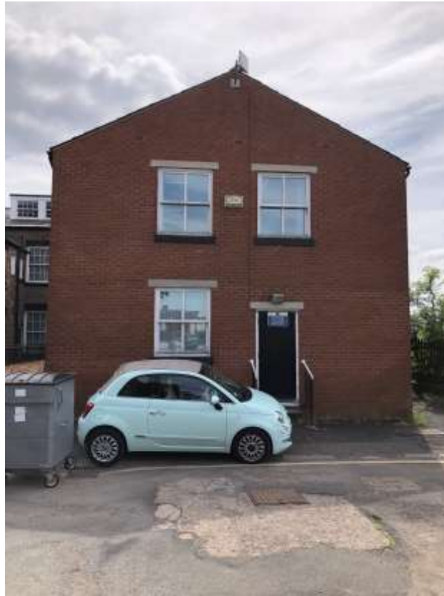
Image 9 – Rear elevation to later extension
