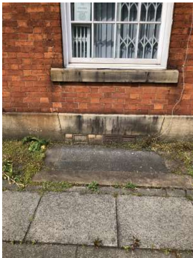
Image 6 – View of infilled cellar grate (No 20)
