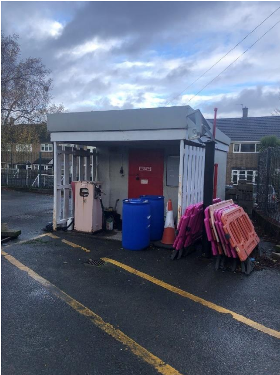
Photograph 9: Building 3 is a storage shed within the training yard. Negligible bat roost potential.
