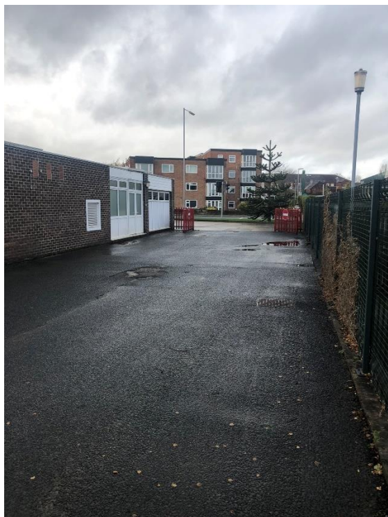
Photograph 5: View looking along northern boundary of the site. North elevation of Building 1.
