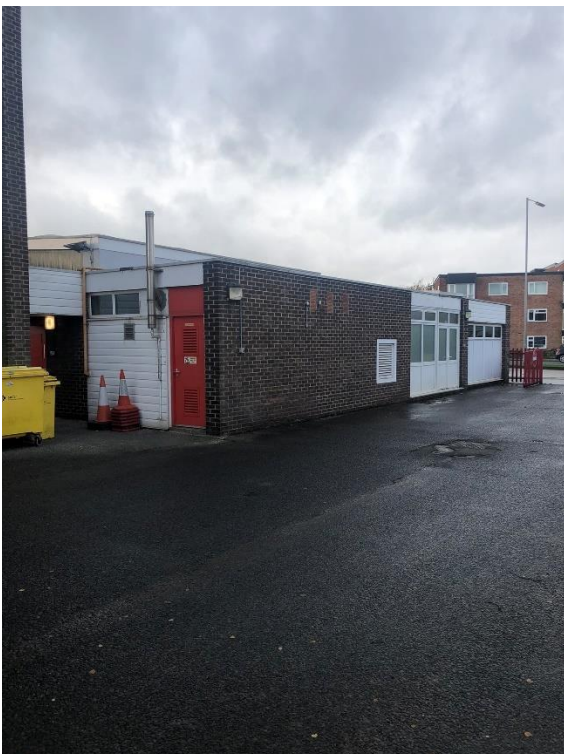
Photograph 10: Building 1, a flat roof single storey brick building. Negligible bat roost potential.
