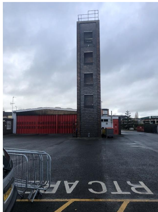
Photograph 7: Overview of the training yard with the training tower in the background.
