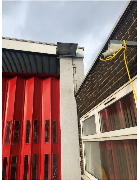
Photograph 11: Close up view of Building 1b and 1c in good structural condition. Negligible bat roost potential.
