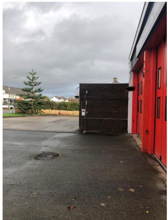
Photograph 4: Front of fire station looking to north west corner of the site.
