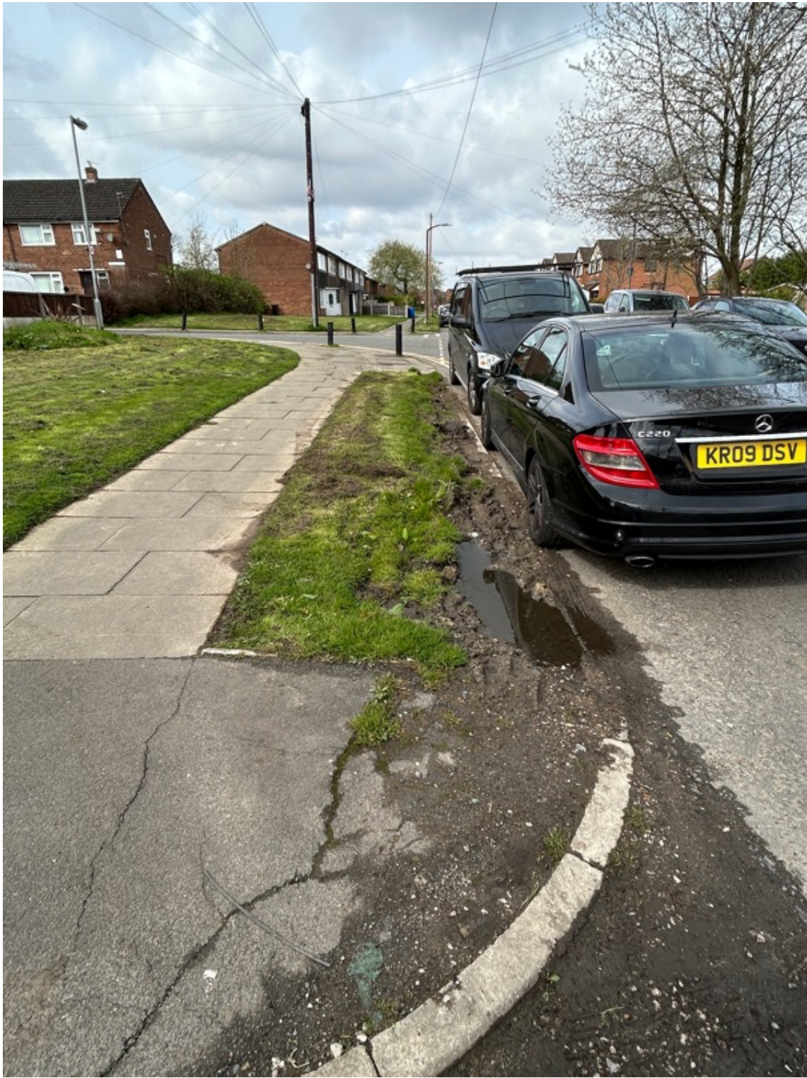
Westminster Avenue – grass verges and footpath
