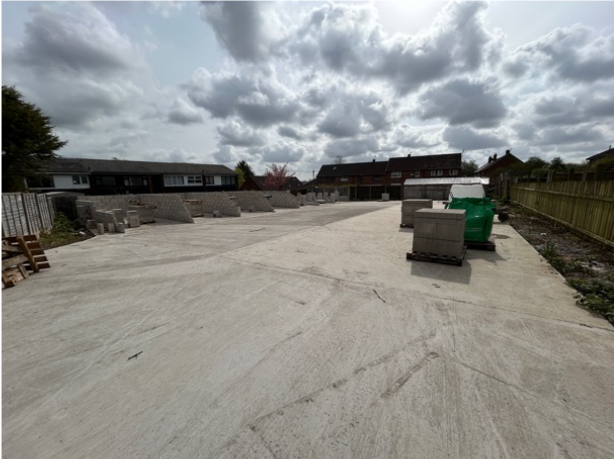
Site – hardstanding – no mud or dust
