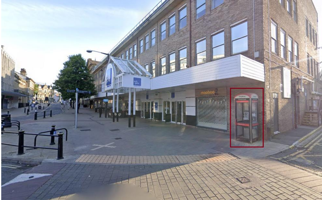
Siting of existing kiosk adjacent the pedestrian crossing point and vehicle accessway
