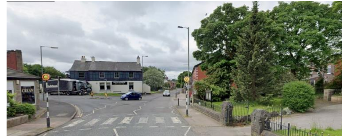
Figure 7b: Existing Holcombe Road junction (reference: 'Google Maps')
