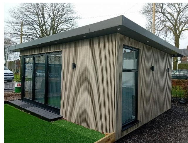
Photo 4: Off-site Building B1 with artificial grass.
