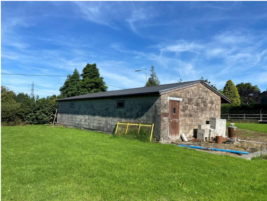
Plate 2 – Character of the exterior of the building on the application site.
