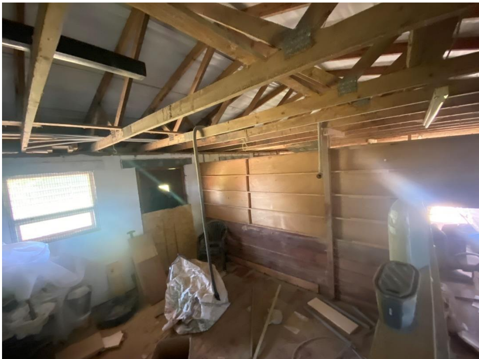
Plate 4 – Further character of the interior of the building.
