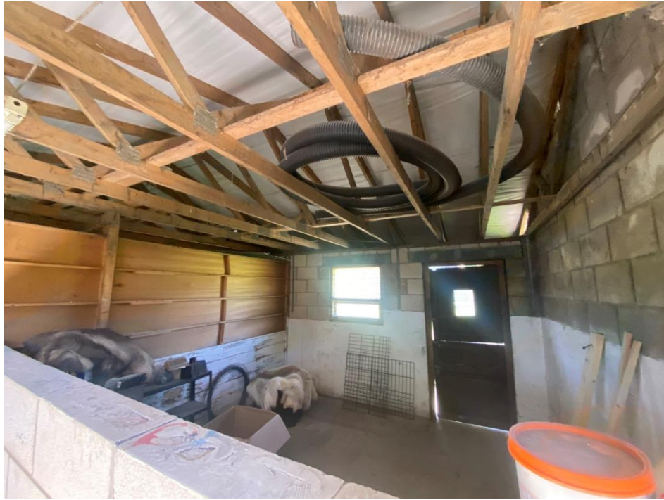
Plate 3 – Character of the interior of the building.
