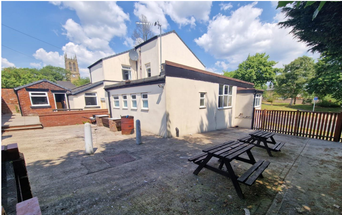
Image 3 – Photograph of southern side/rear elevations of building and large enclosed yard area
