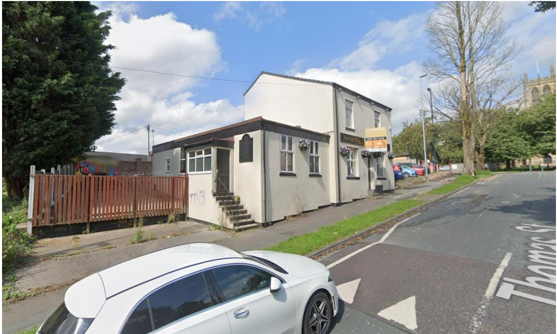
Image 2 - Streetview image of vacant former public house (with marketing board visible) taken from Thomas Street facing north west (dated April 2023). This image shows the side/rear external staircase and entrance that will be demolished as part of the development proposal.
