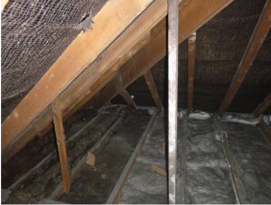
P1 Loft 1, insulated floor, felt lining
