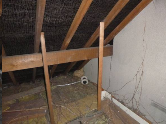
P2 Loft 2, insulated floor, felt lining
